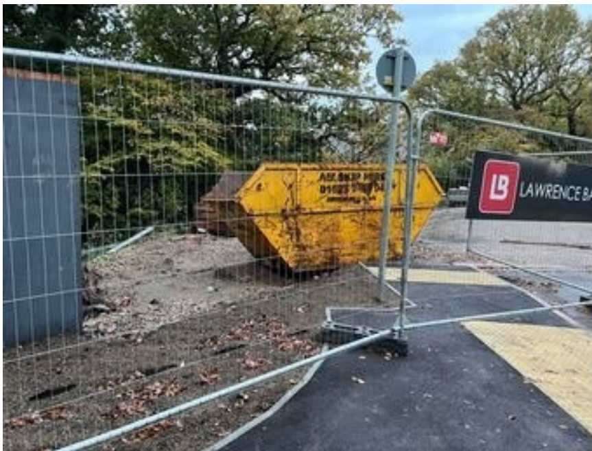
Figure 3: Street view of the entrance of the site on 21 October 2025
