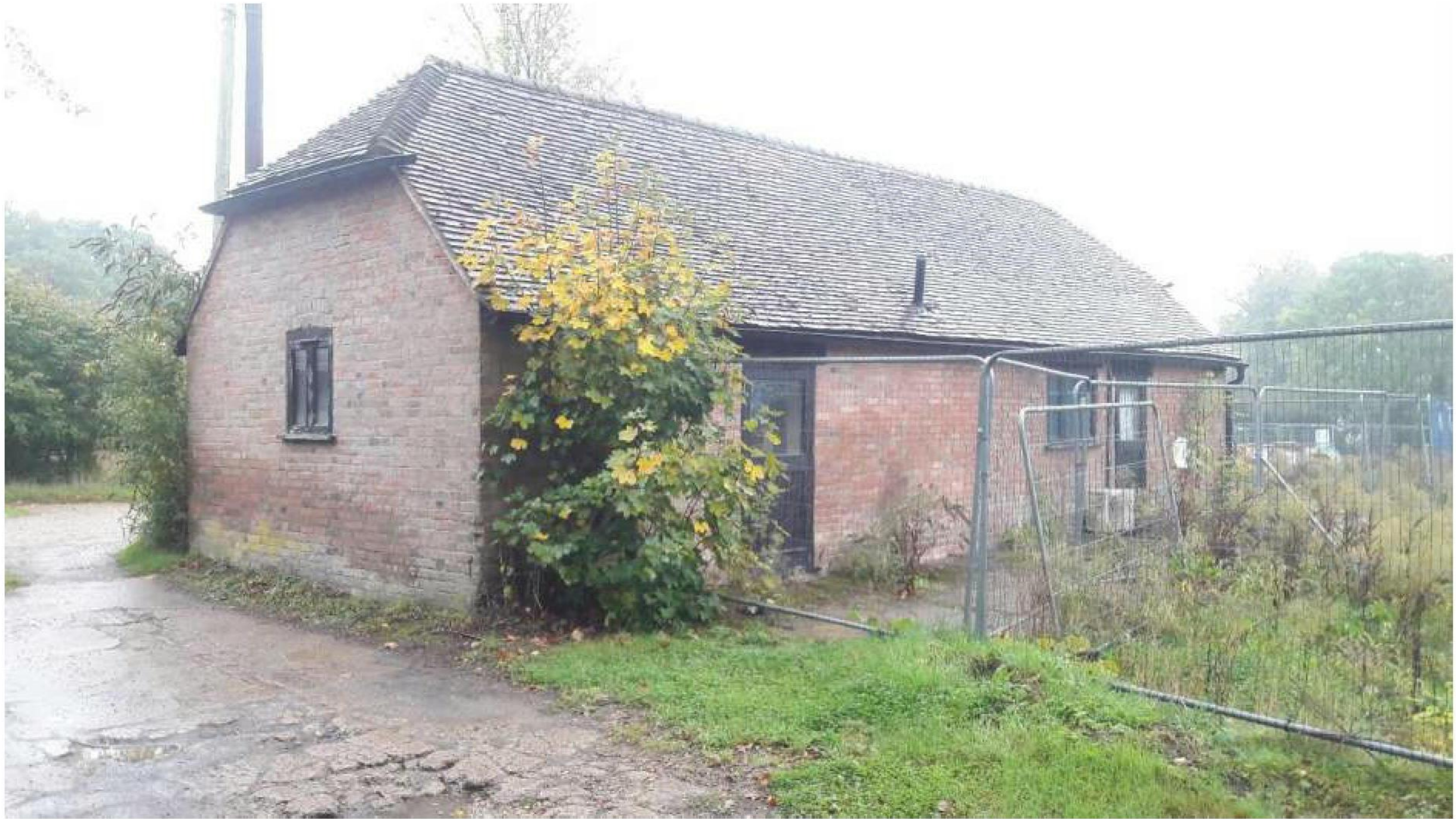
Plate 11: The Old Dairy, facing south-east.
