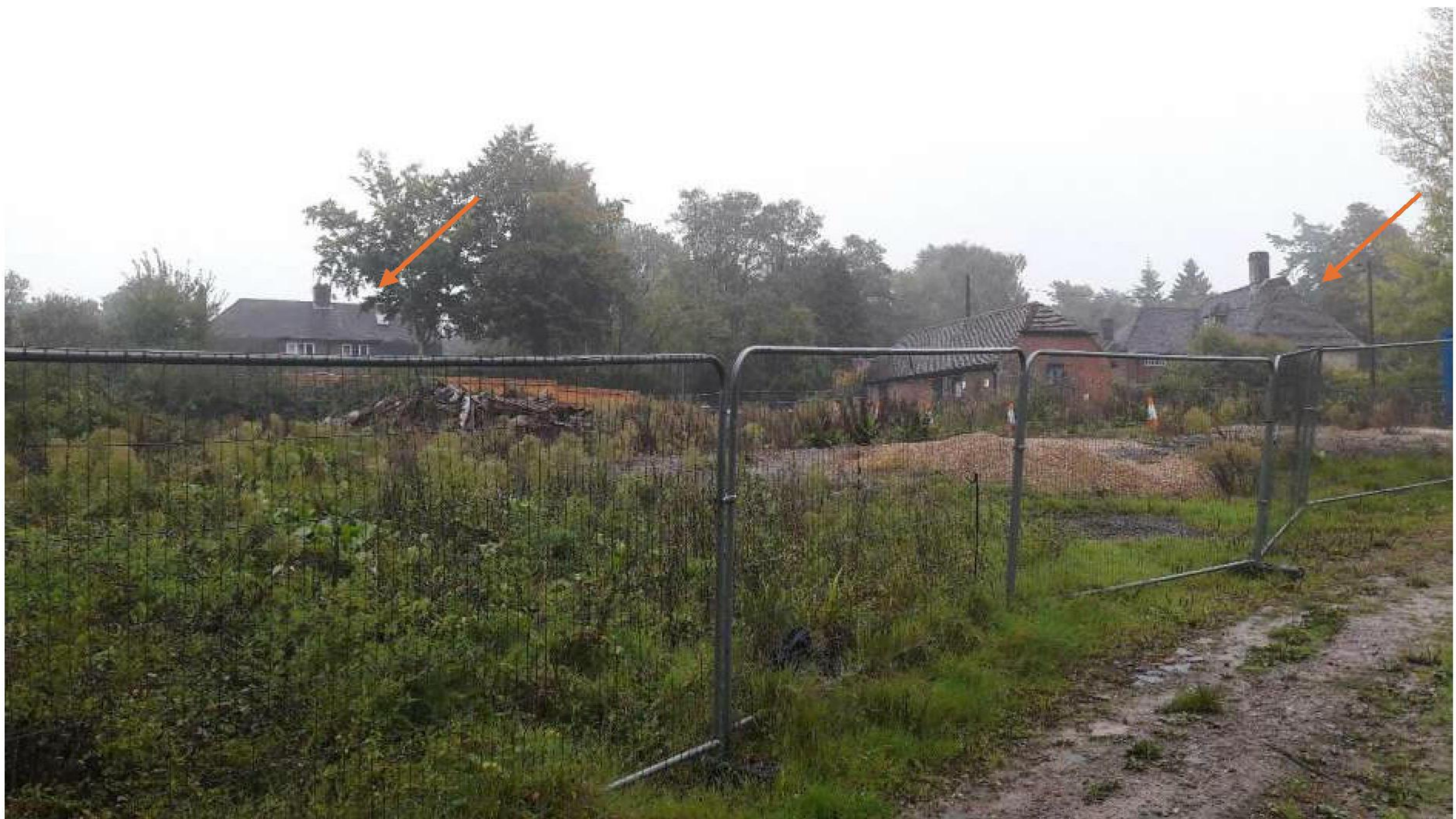
Plate 4: Looking north/north-east across the southern part of the Conservation area, showing the buildings of Townhouse Farm. East Cottage (left) and Townhouse Farmhouse (right) are indicated.
