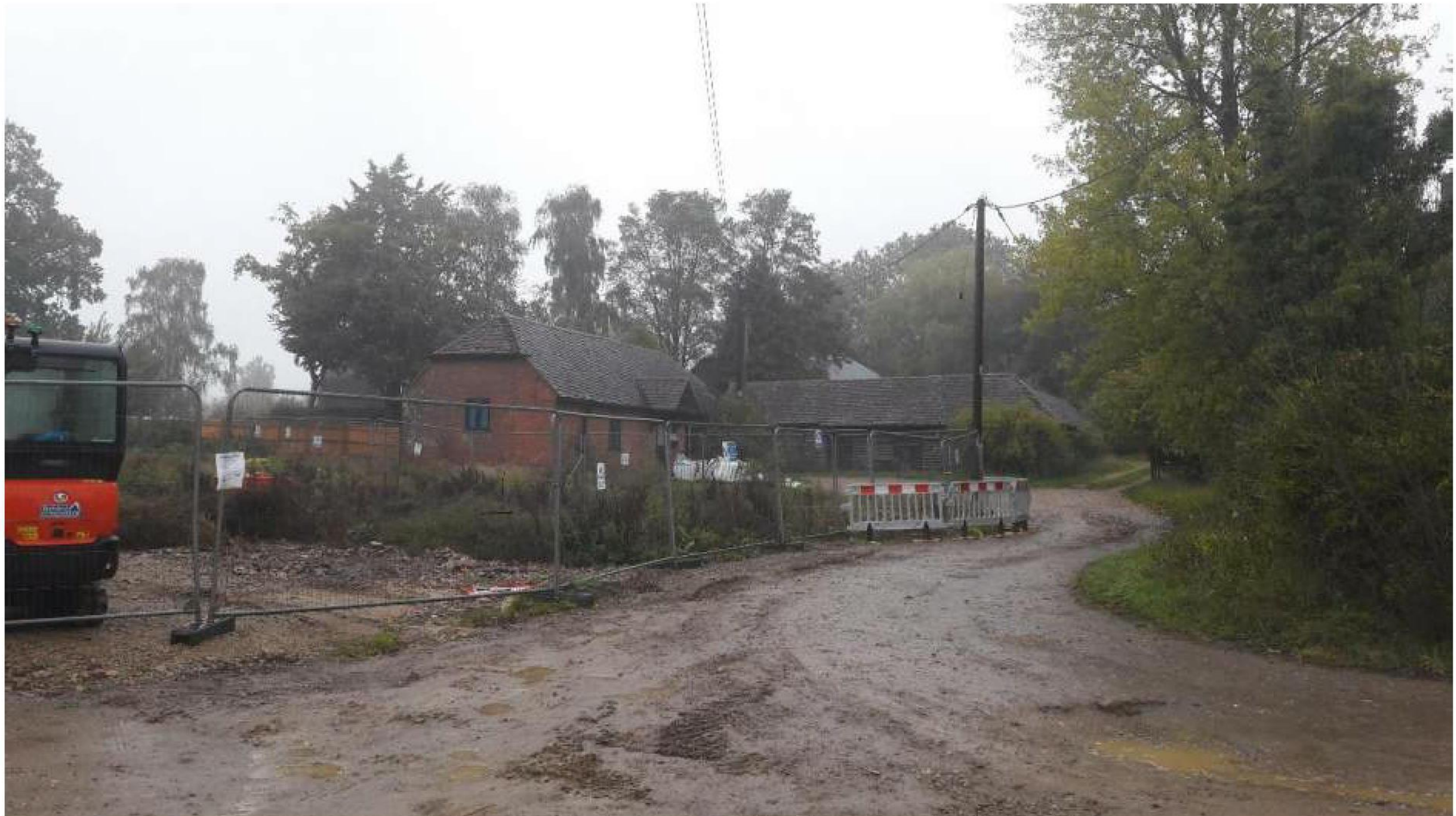
Plate 3: The southern part of the Conservation Area, facing north-west, showing the buildings of Townhouse Farm.
