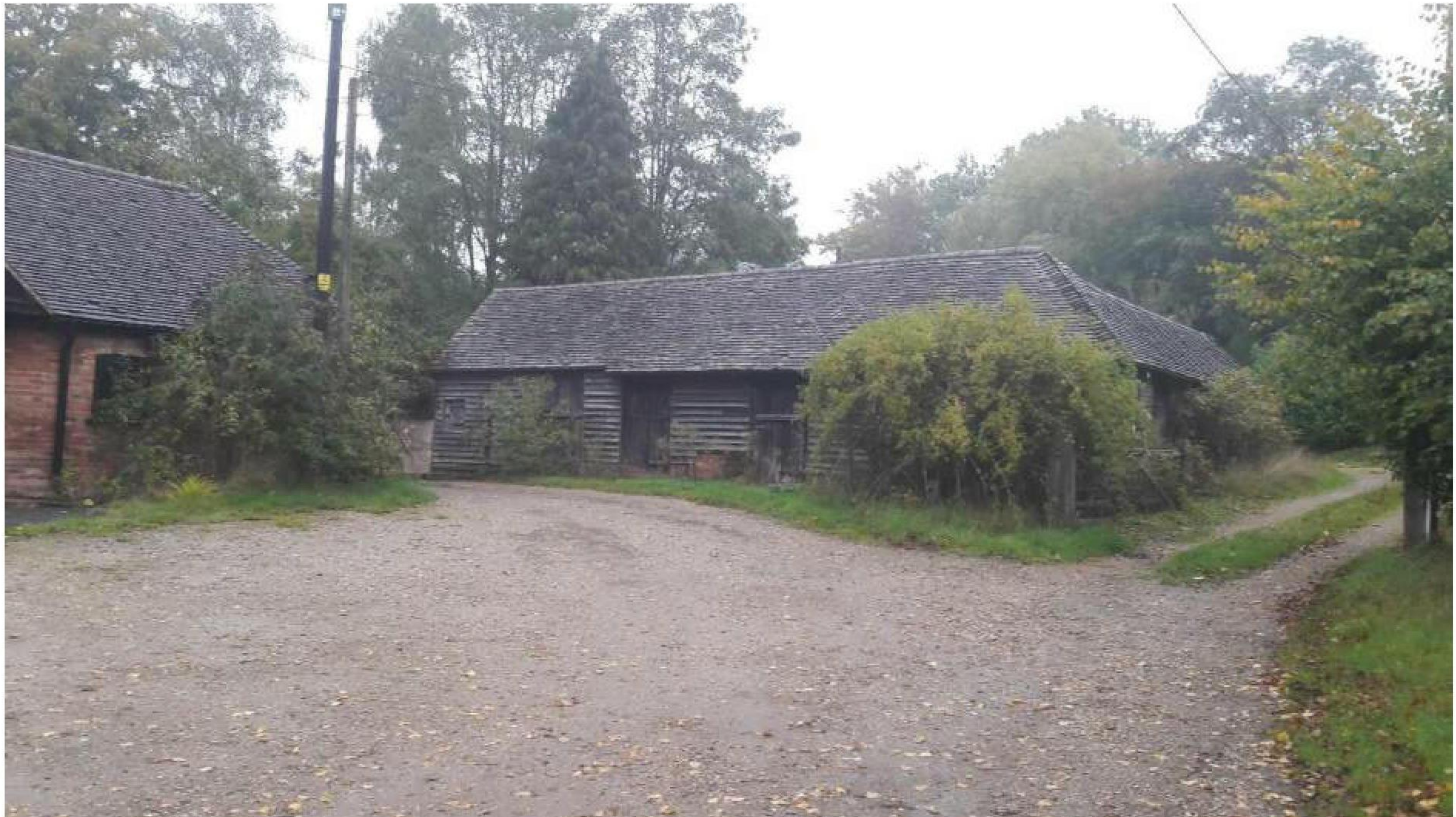
Plate 9: The stable west of Townhouse Farmhouse, facing north.
