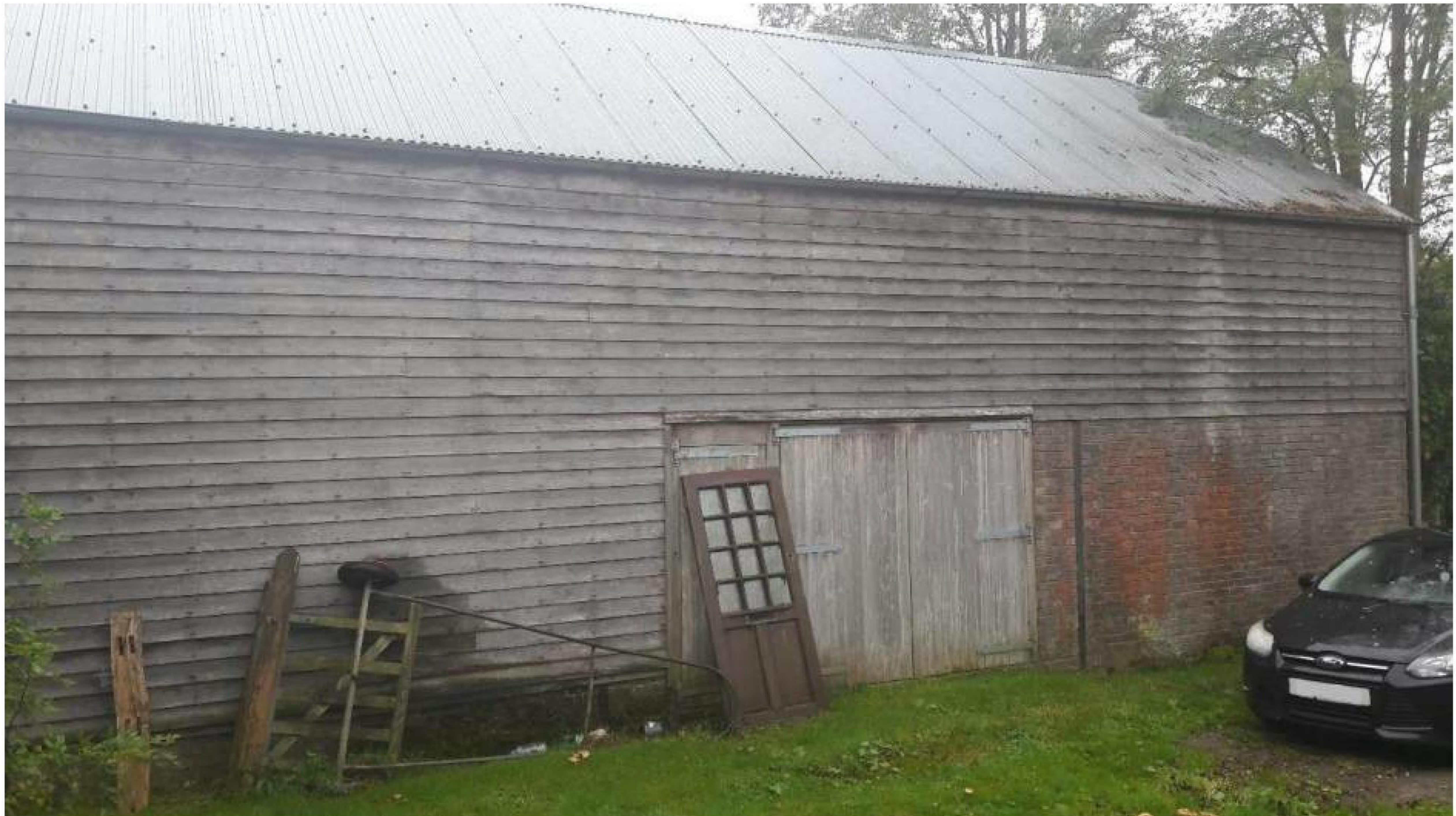
Plate 7: The barn north-west of Townhouse Farmhouse, facing south-east.
