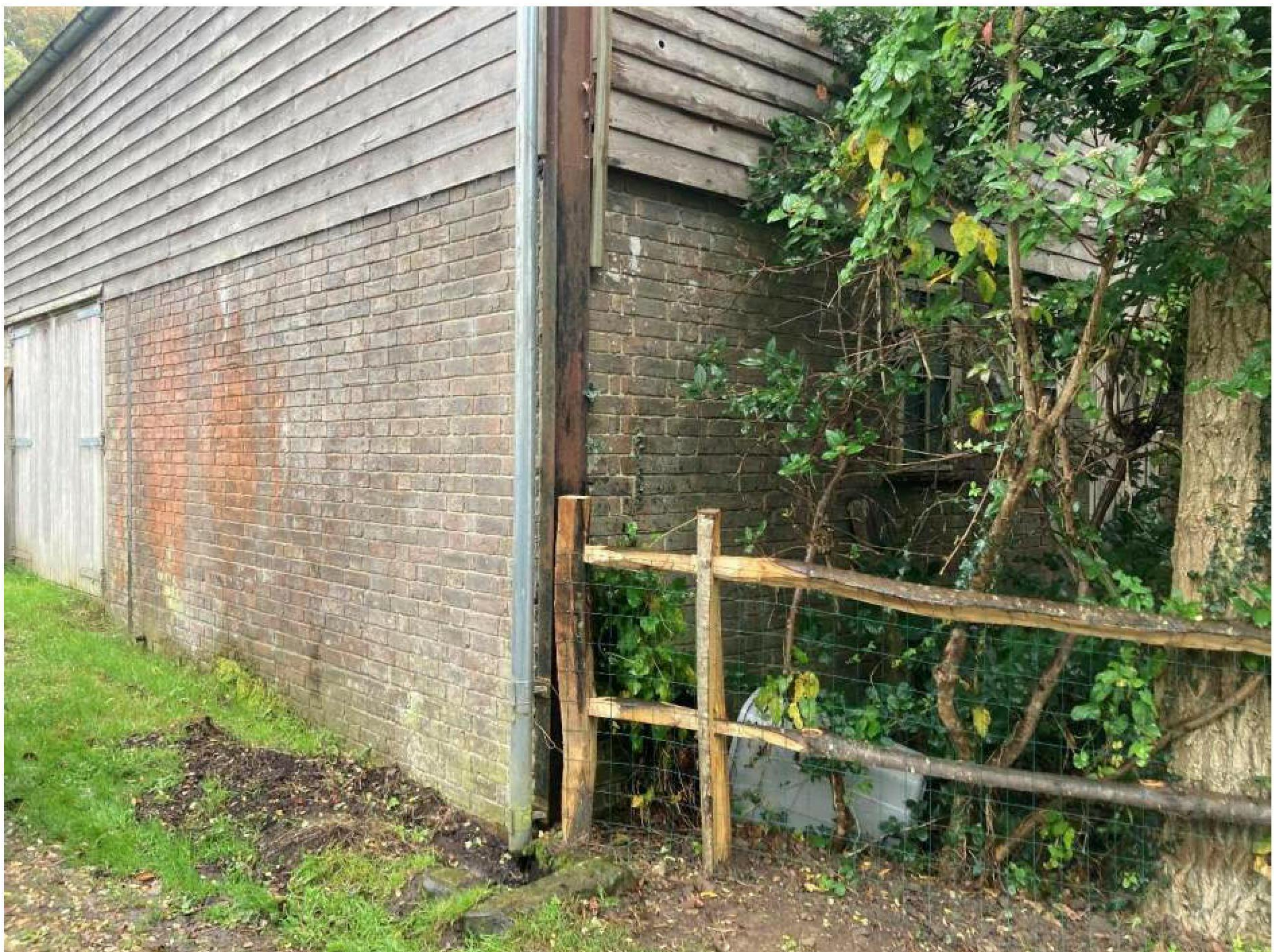
Plate 8: The south-west corner of the barn showing iron girders used in its construction.
