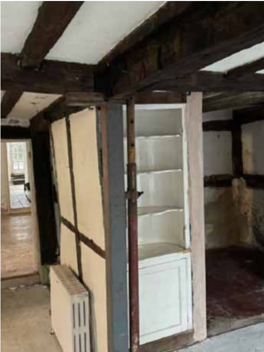
Pre-construction photograph - steel post supporting timber frame
