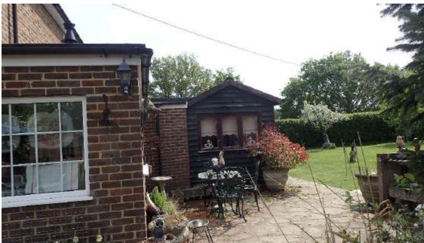
Photograph: Concrete Paving Rear Garden
