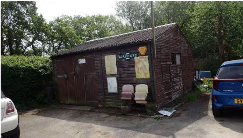
Photograph: Tarmac parking and site access around Garage
