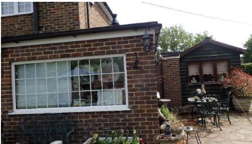
Photograph: Concrete Paving Rear Garden
