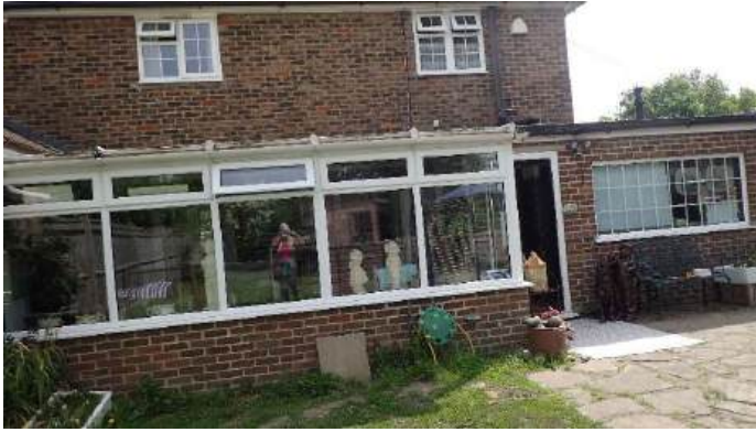
Photograph: Concrete Paving Rear Garden
