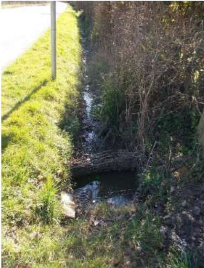
Photograph: Drainage Ditch and Trash Screen Inlet
