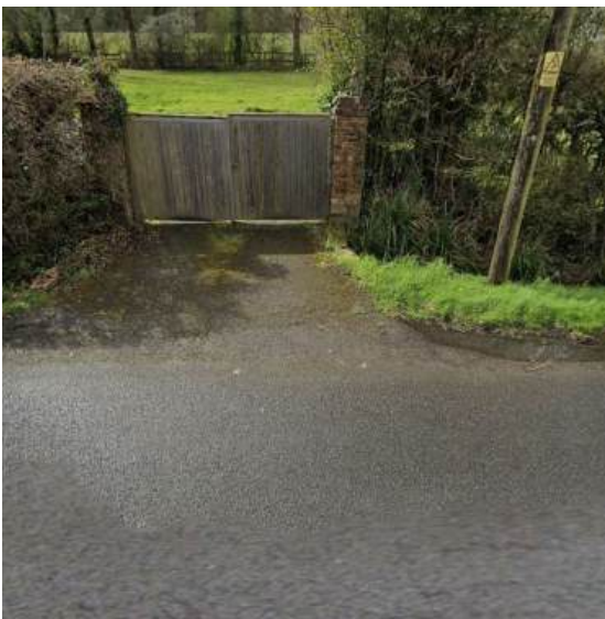
Photograph: Tarmac site access and vehicle crossover
