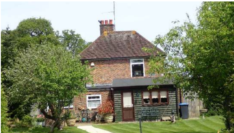
Photograph: Concrete Paving and footpath Side Garden
