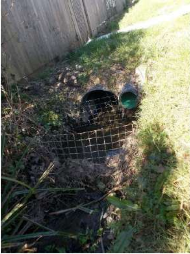
Photograph: Drainage Ditch , Culver Inlet and Trash Screen
