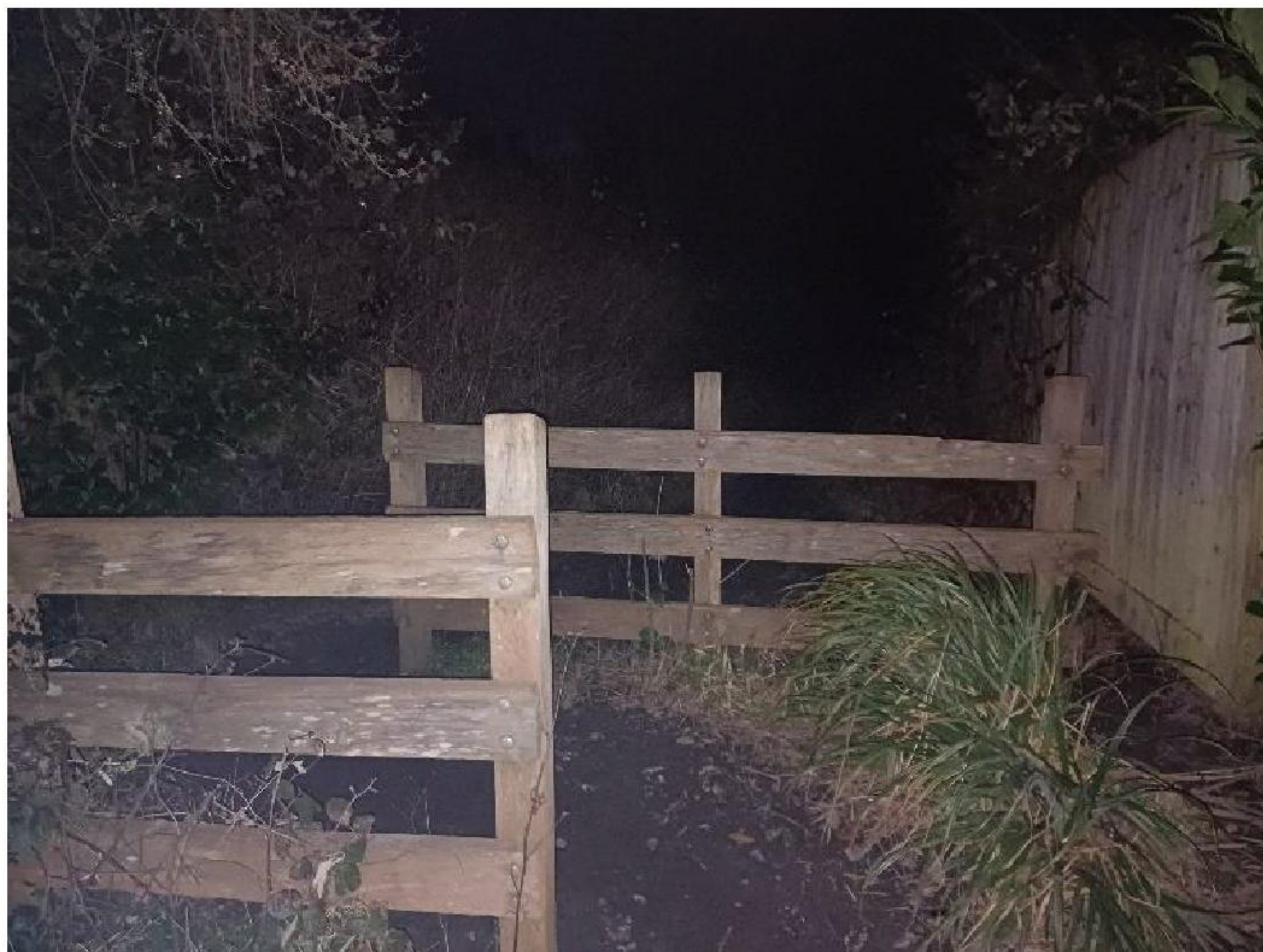
Figure 5: Uneven sections of 29CU footpath
