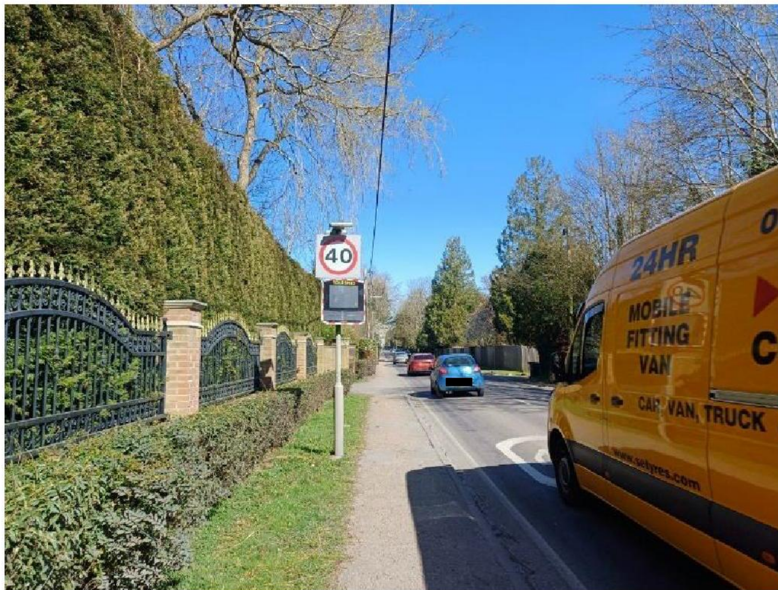
Figure 1: Vehicle-Activated Sign installed on A272
