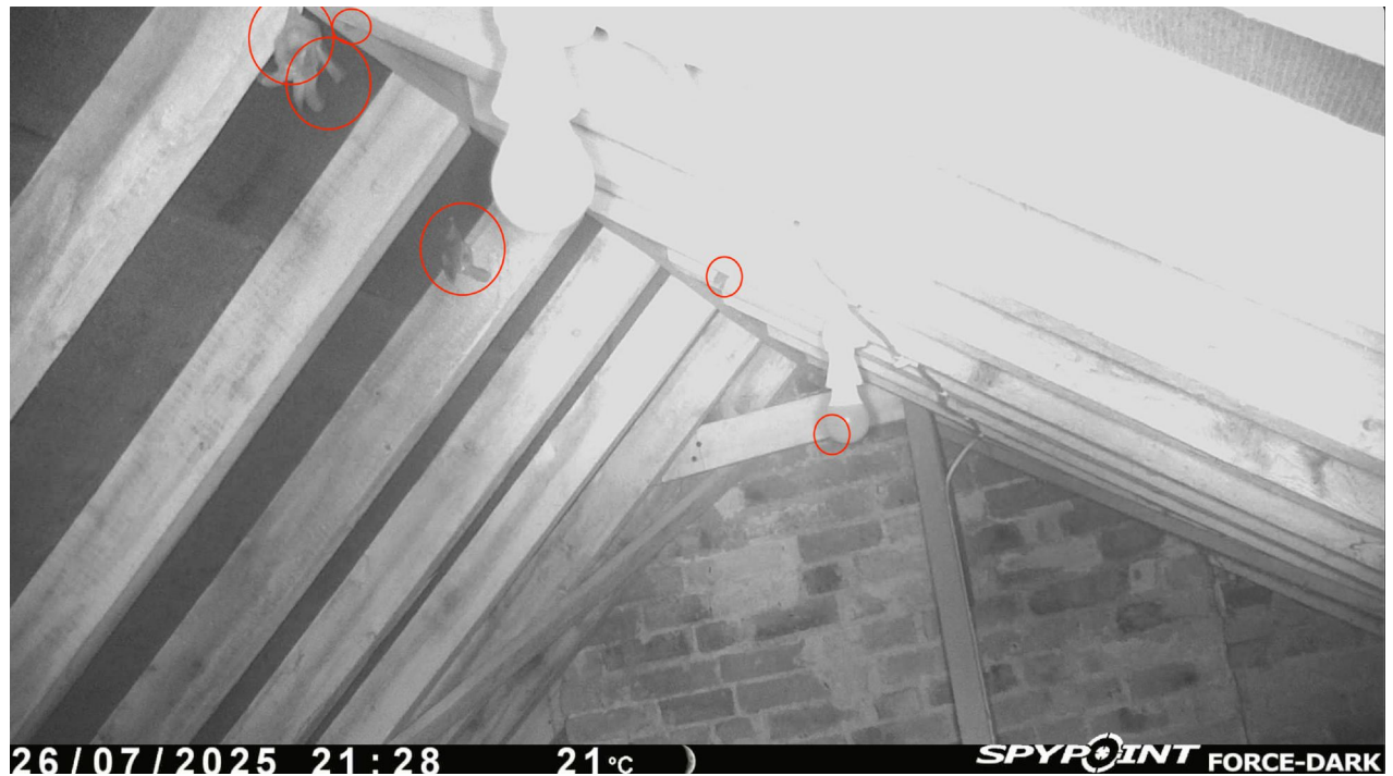
Figure 1. Screenshot from the Spypoint trail camera on 26 July 2025 21:28 showing six brown long-eared bats roosting separately on bitumen felt (red circles).
