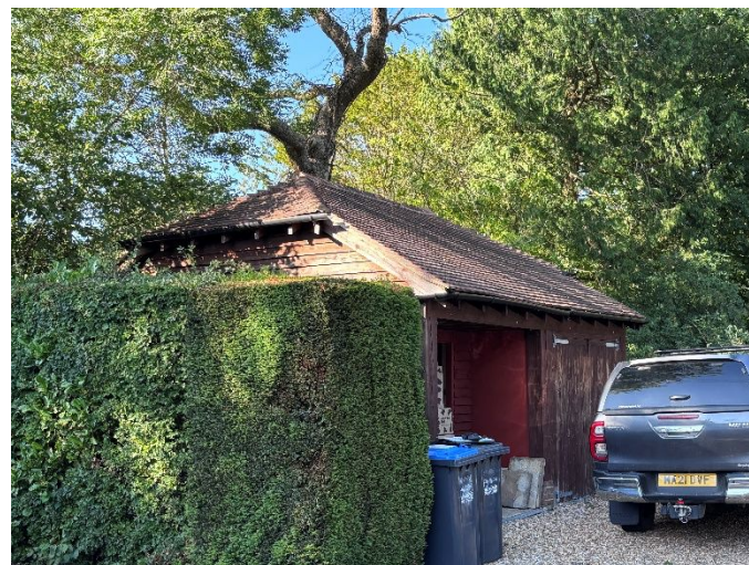
Photograph 4. Western and southern elevations of the garage.
