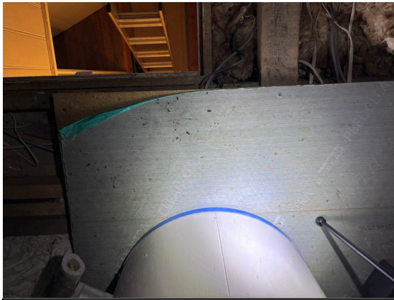
Photograph 1. Six bat droppings visibly identified as long eared bat droppings on the floor under the ridge.
