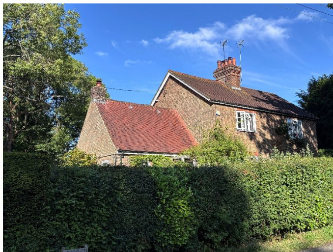
Photograph 1. Northern and western elevations of the property.
