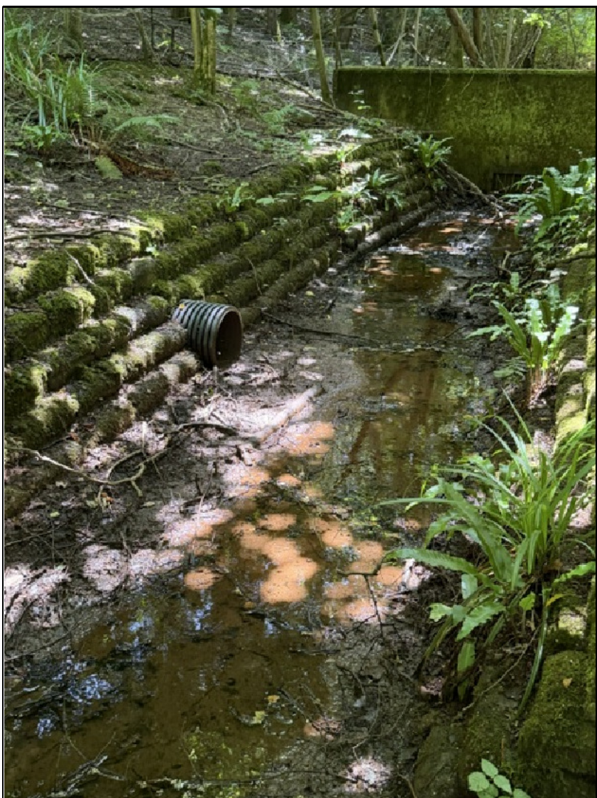
Substantial 'Bagwork' channel leading to concrete culvert headwall. 300mm dia side connection
