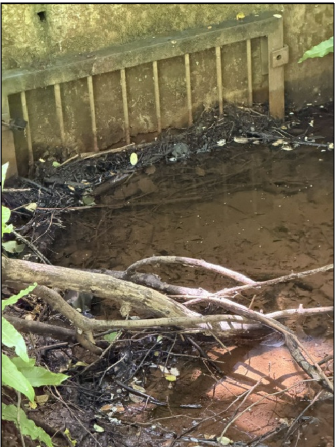
Culvert Pipe with Grille Estimated 600mm diameter minimum Requires clearing
