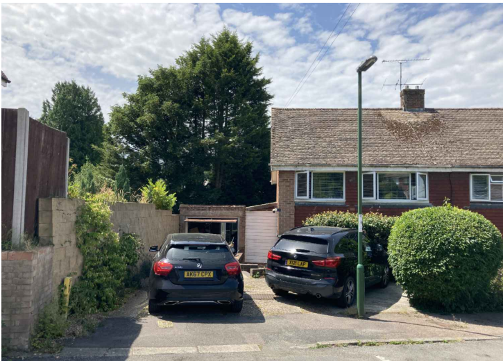
Photo 2: Existing front elevation
