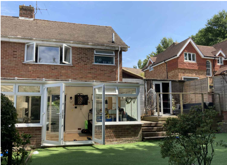
Photo 3: Existing rear elevation
