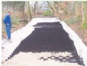
CellWeb during installation.
