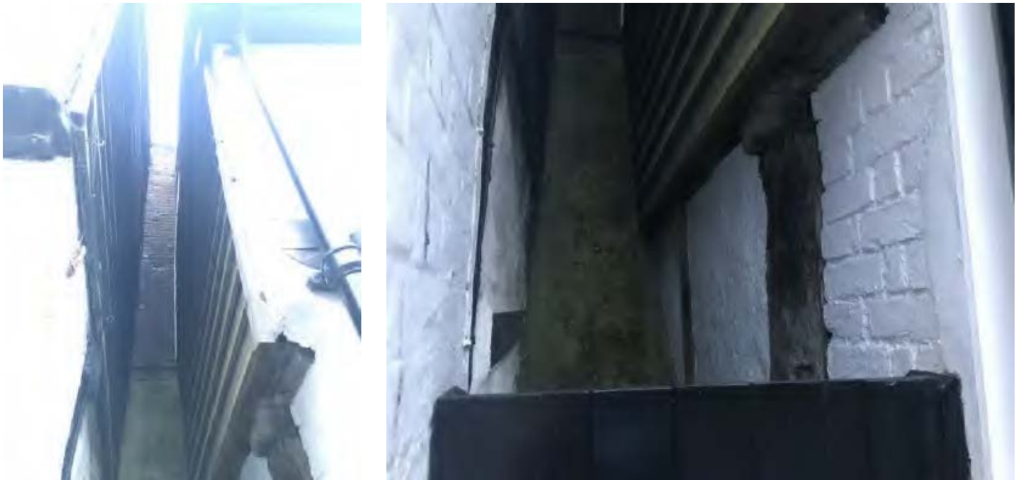
Recent photographs of timber weatherboarding
