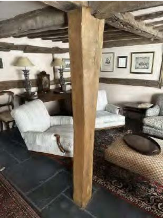
Steel post replaced with traditional gunstock post in seasoned oak
