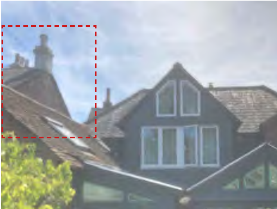
109 High Street south gable wall before re-rendering
