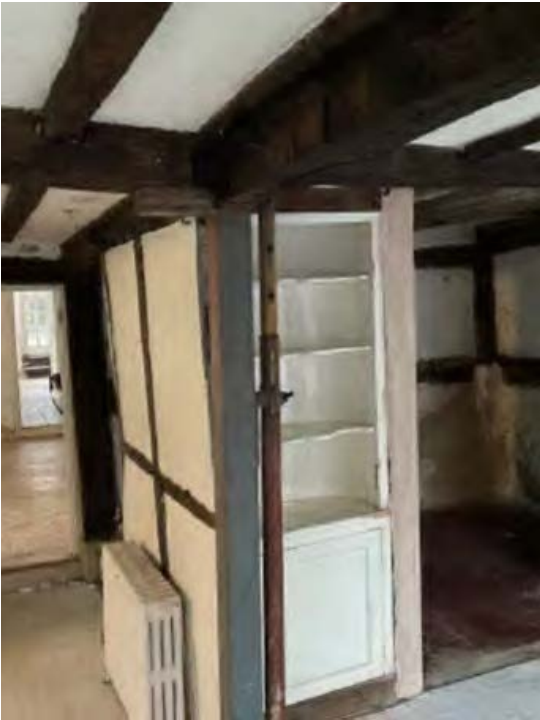
Pre-construction photograph - steel post supporting timber frame
