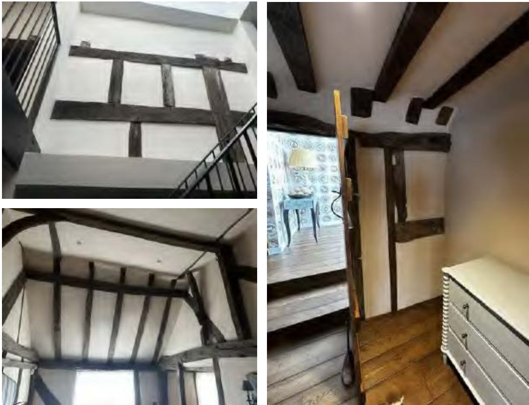
Photographs of restored historic oak frame
