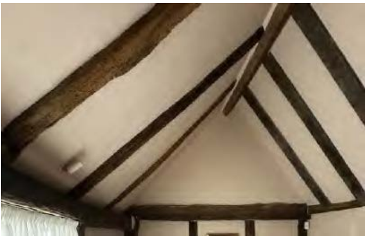
Vaulted Ceiling in SE Bedroom
