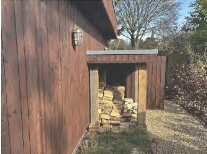
Current photograph- garage
