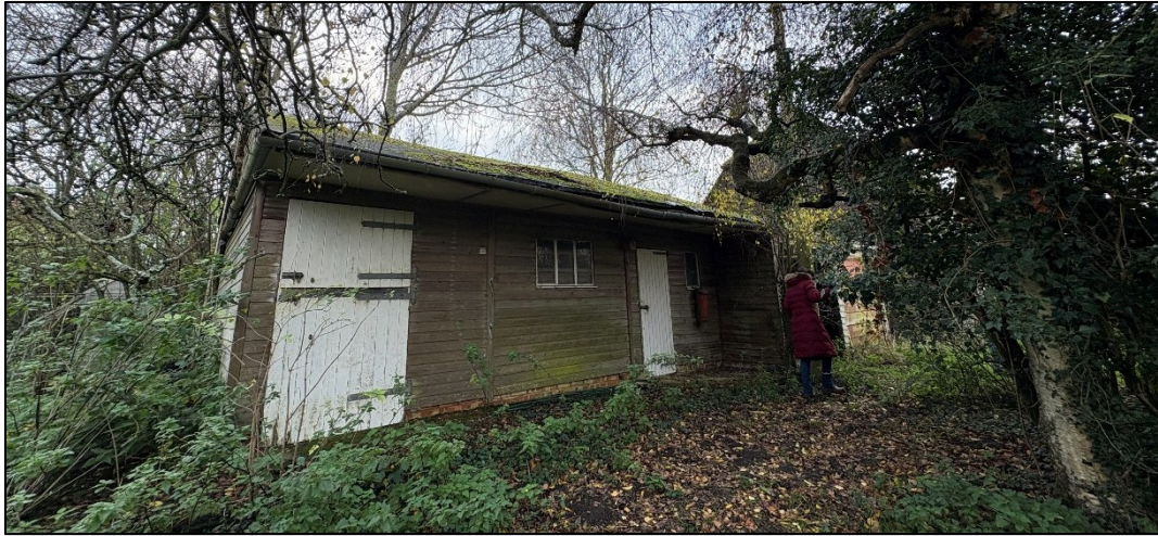
Figure 5: Existing timber outbuilding to west of barn
