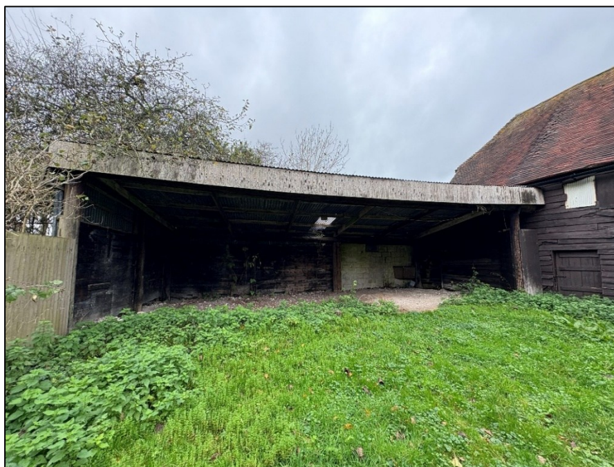
Figure 4: Existing extension to west of barn
