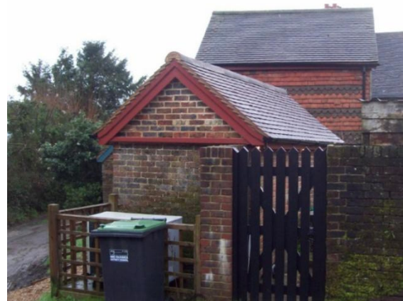
Figure 5 - Existing West Elevation outbuilding
