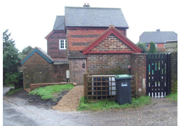
Figure 7 - Existing West Elevation outbuilding
