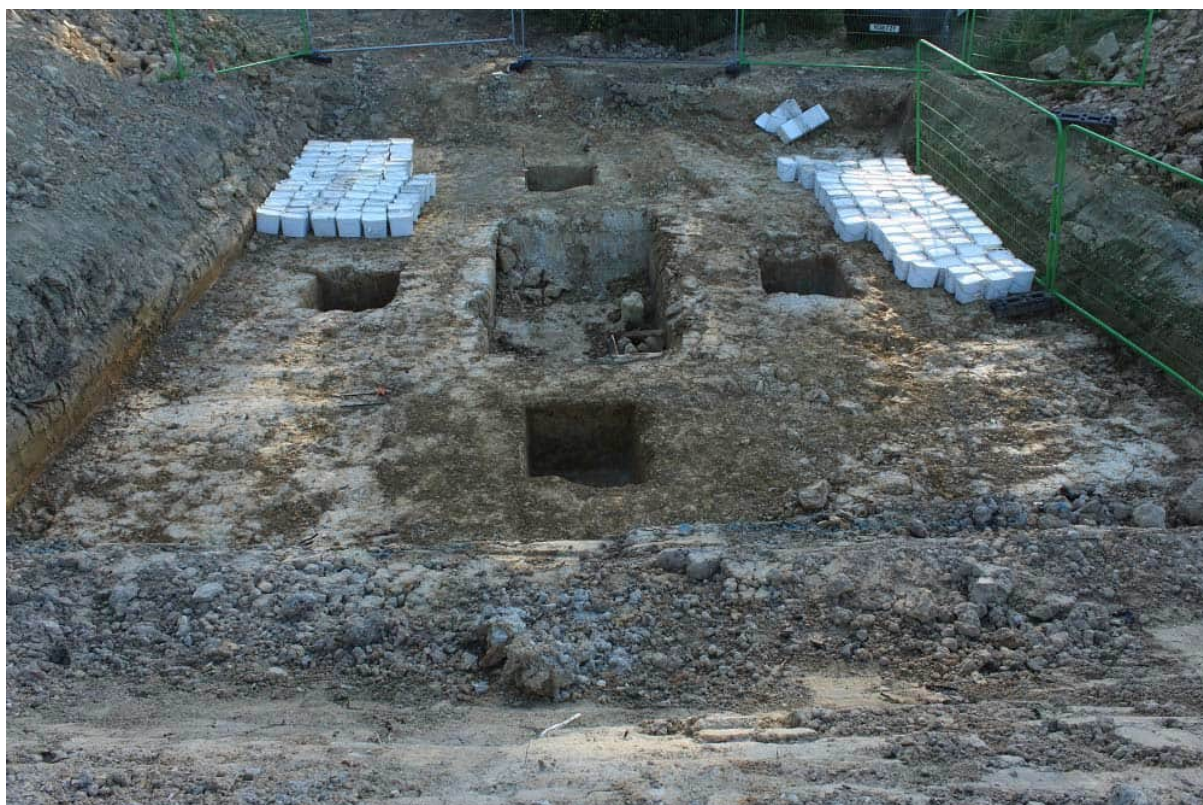
Plate 10. Test pits in area 2, view east
