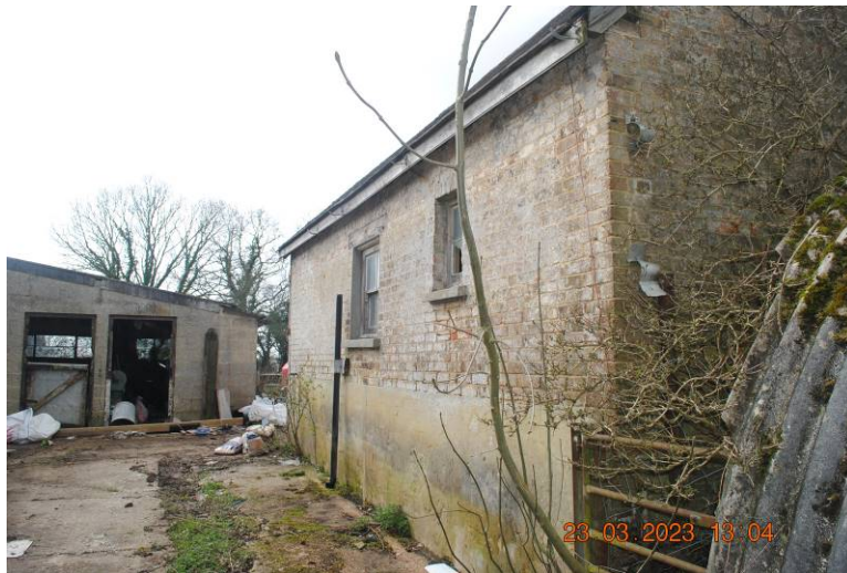
Photograph 1: A view south towards the storage building being converted. The building is situated in an existing yard comprising hardstanding which extends in all directions.
