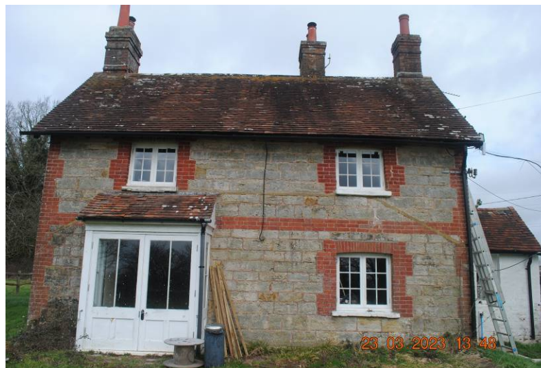
Photograph 4: Looking north towards the farmhouse. The patio will extend along this elevation.
