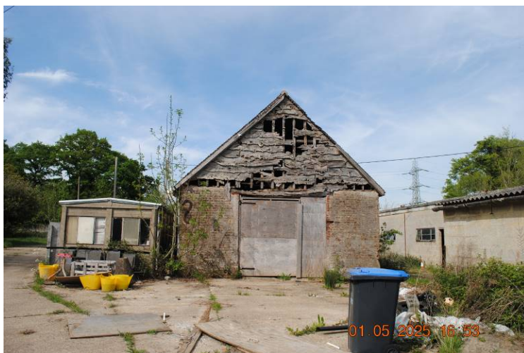
Photograph 2: A view east towards the storage building.
