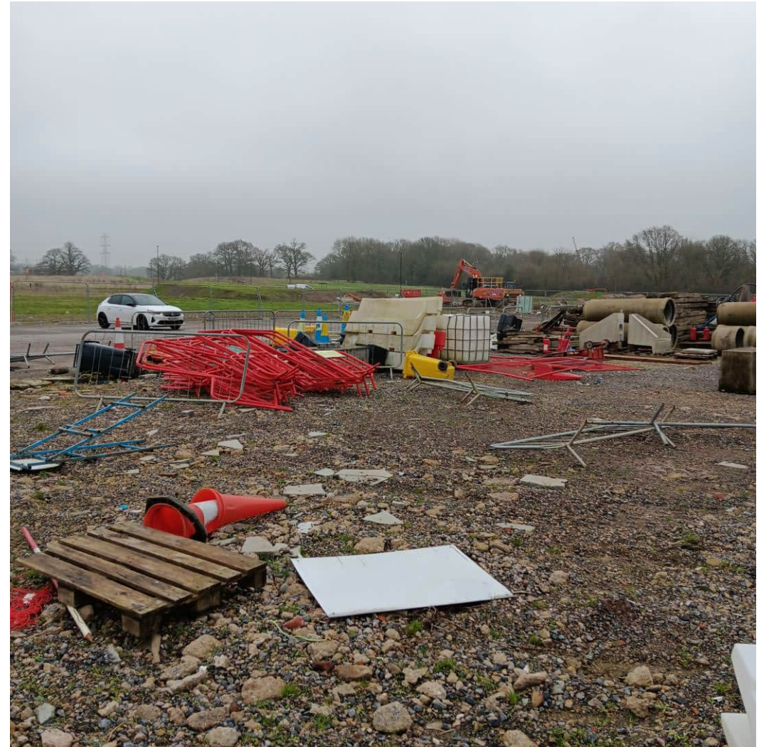
Photograph 2: Site compound area
