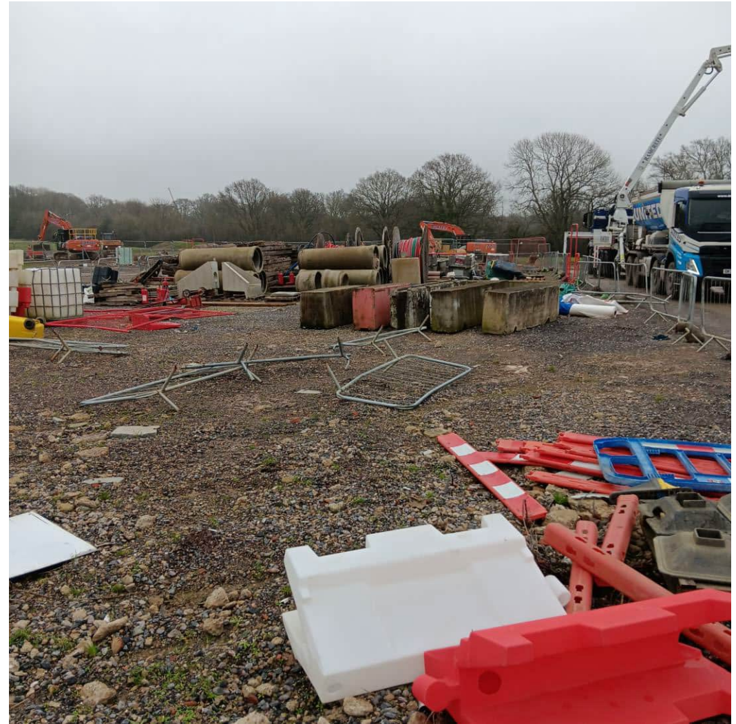
Photograph 4: Materials Storage in compound area
