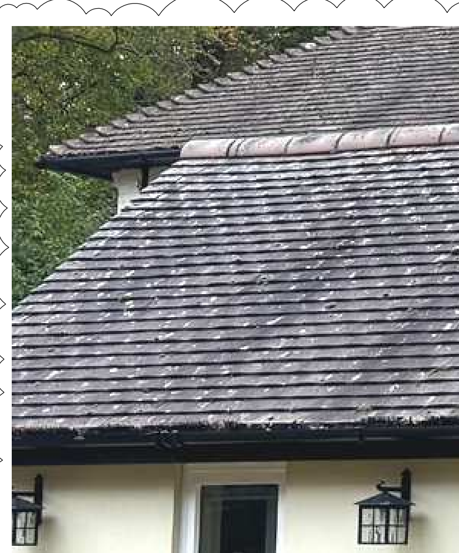
Existing tiles to be re-used.
