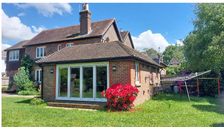
Figure 2 – Existing house with plot for extension on the right had side
