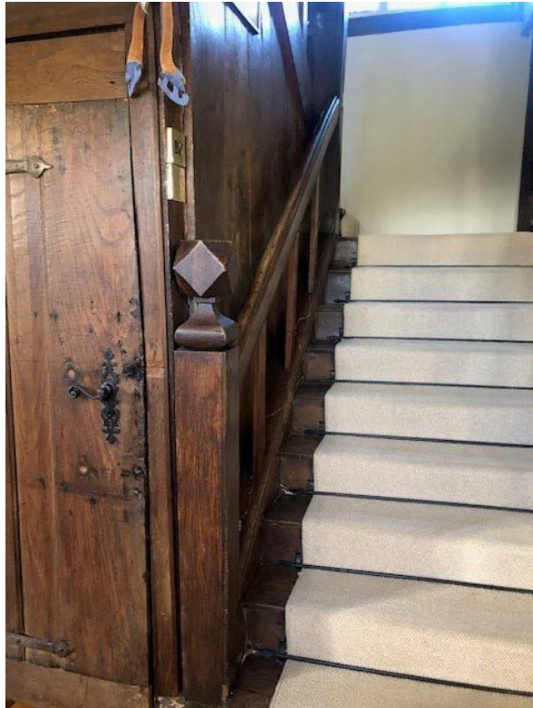
New joinery timber to match existing.
