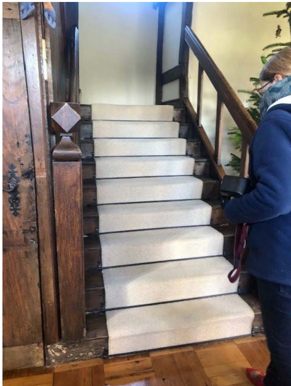
View of Stairs
