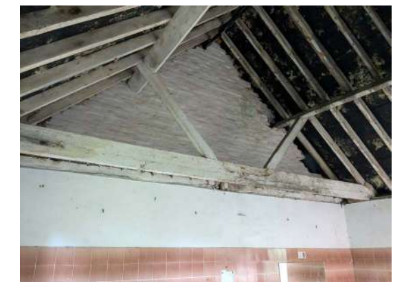
Example of slim bottom chord in south-east range
