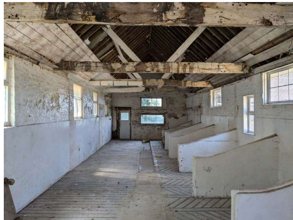
Existing view looking west of south-west range, note sloped floor.
