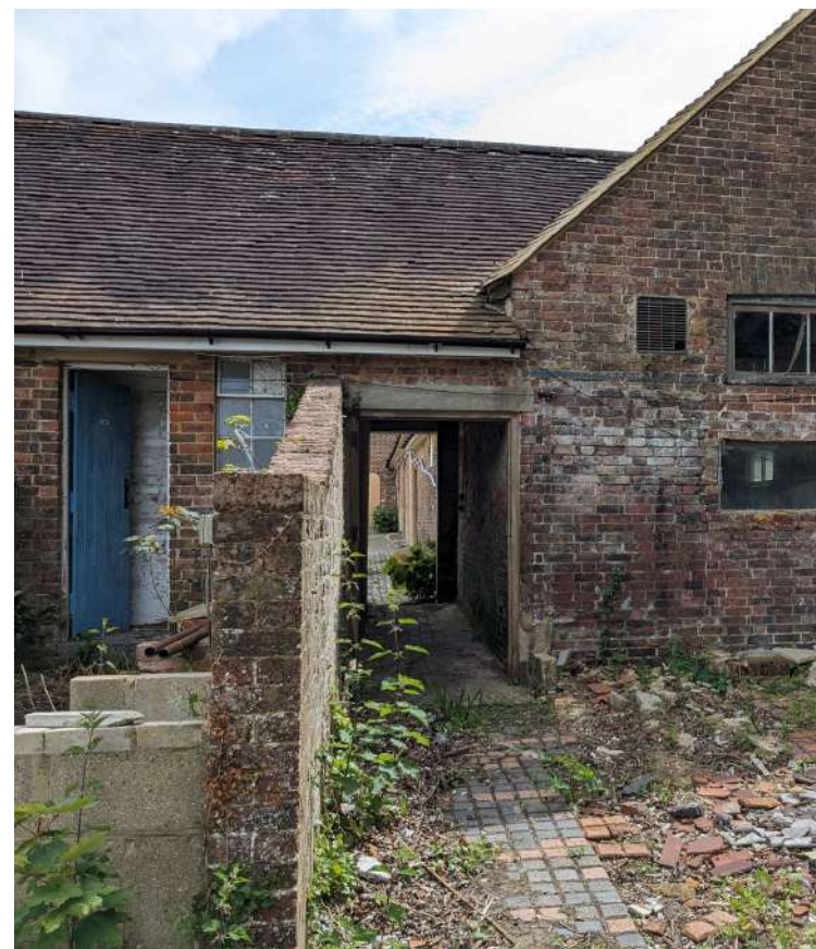
West passageway entrance into courtyard
