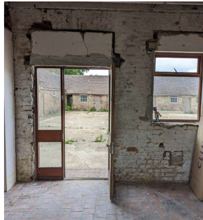
View from east range stable over farmyard
