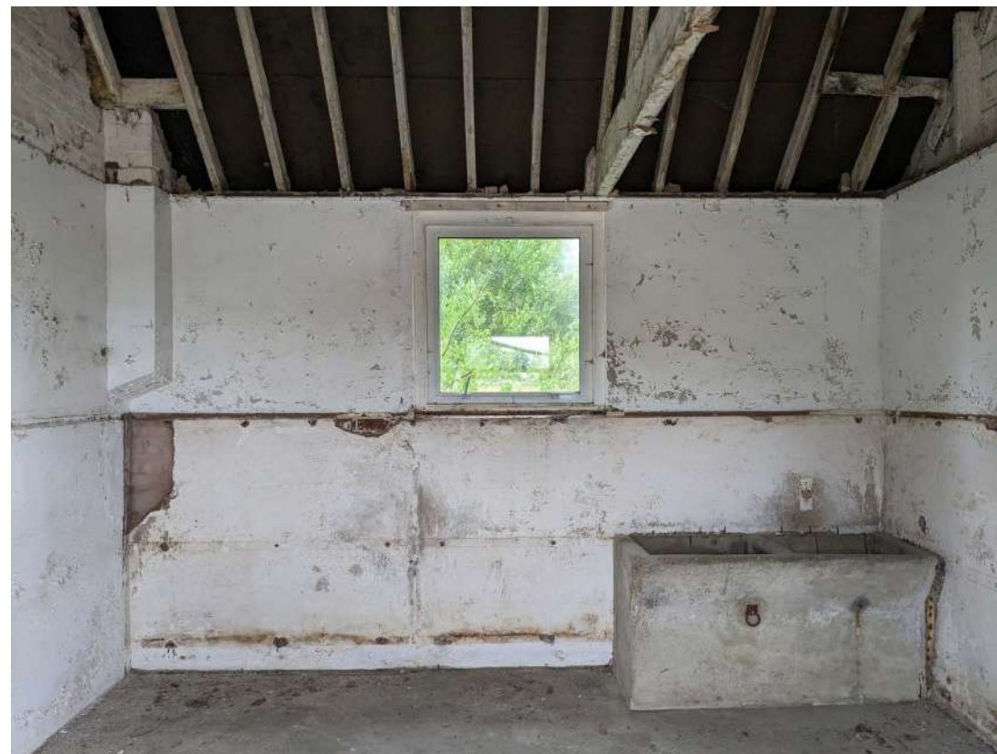
View within south range stall looking into garden, concrete trough within corner
