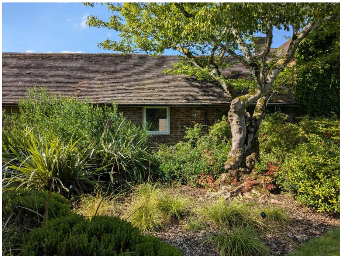
View looking north of the south range from Wakehurst gardens
