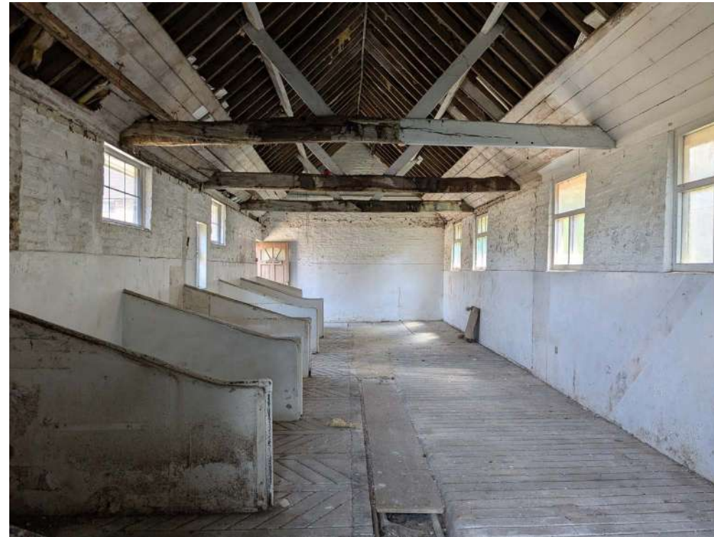
Existing view looking east of south-west range, note sloped floor.
