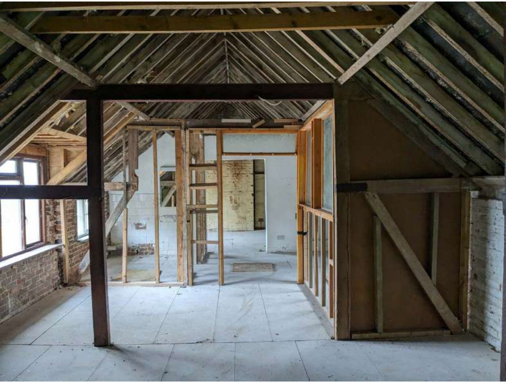
First floor view looking north
