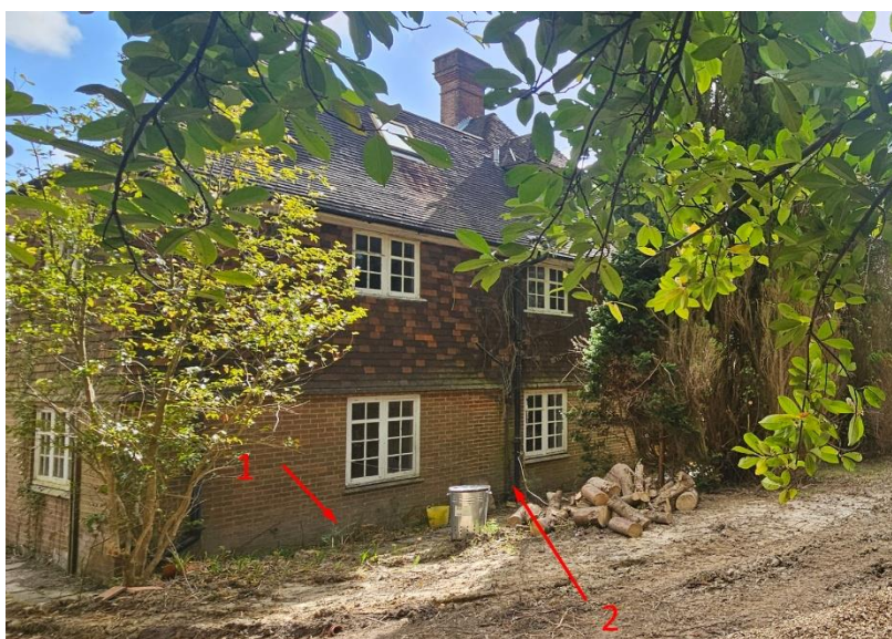
Figure 19: Image to show where each air brick is located
