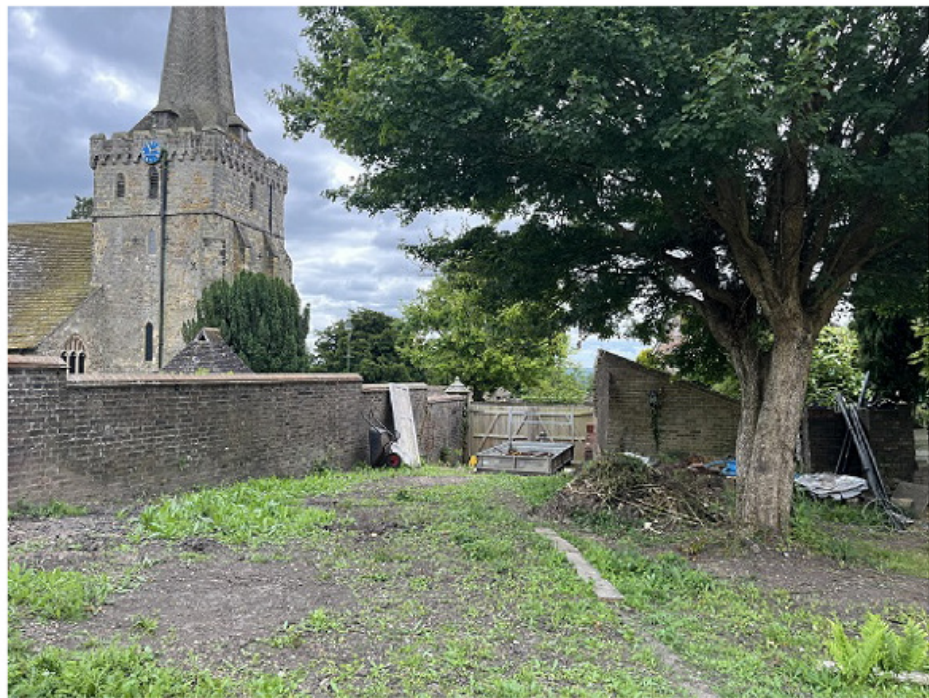
existing brick walls to be retained
