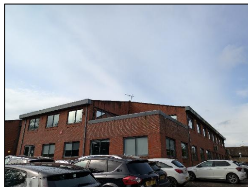
Figure 5: Sussex House building
