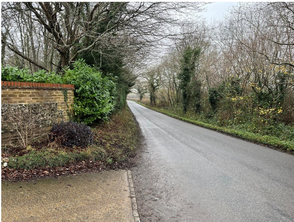
Photo Above: The Existing Visibility Splay to the North
