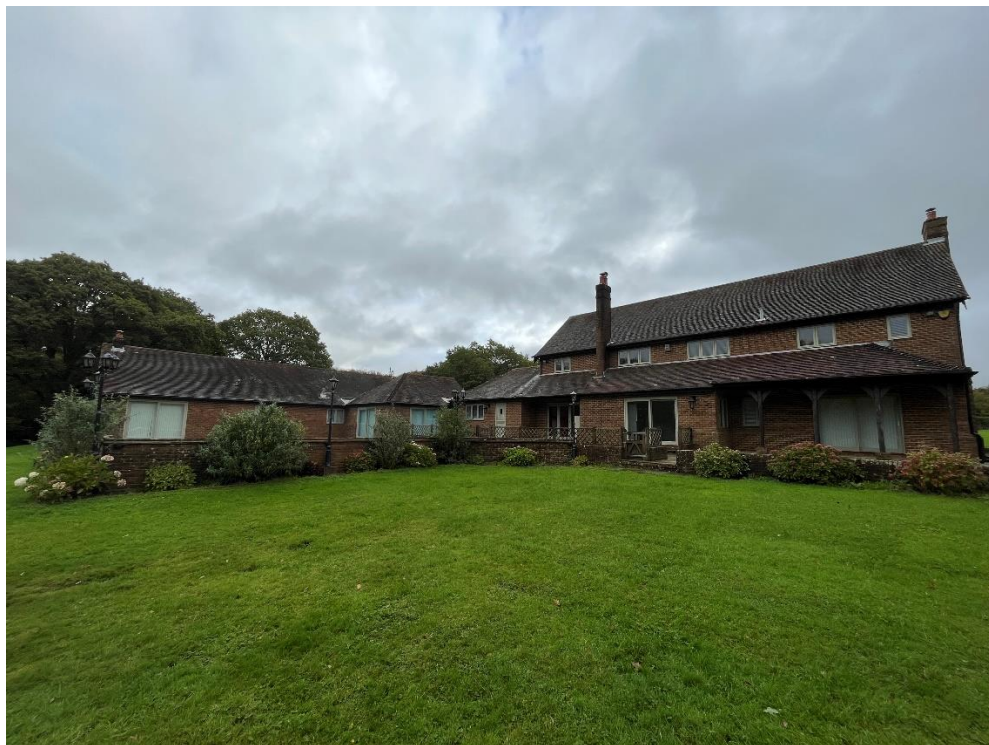
Photo Above: The existing dwelling at East Wood Farm
