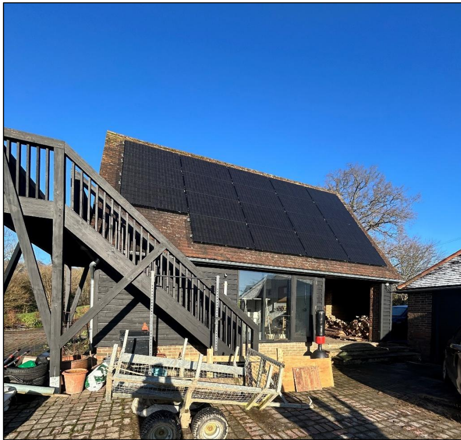
Figure 2: Photograph of southern elevation of workshop building showing solar PV panel array.
