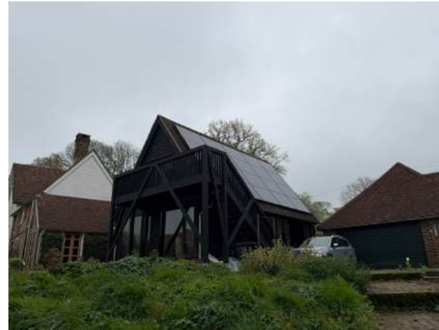
Plate 5 View towards southern end of the listed building (left) and workshop (centre) showing solar panels to roof.
