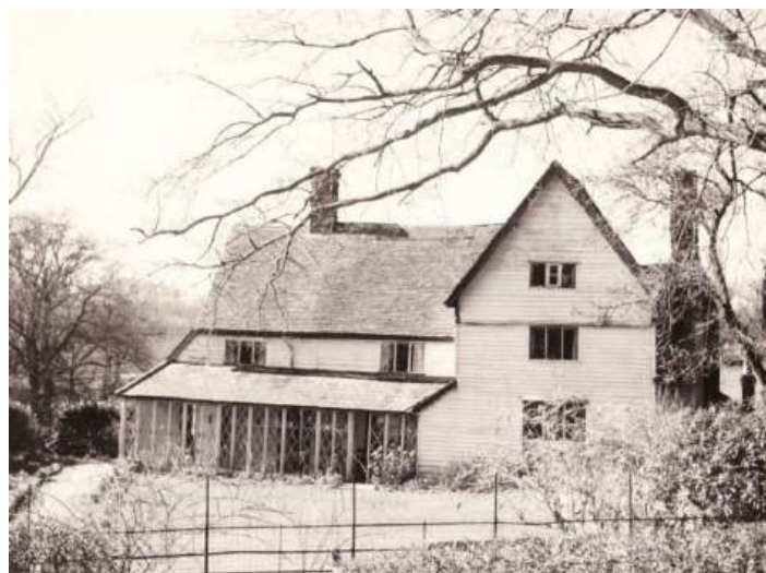
Figure 10 1970s showing eastern elevation of the farmhouse.
