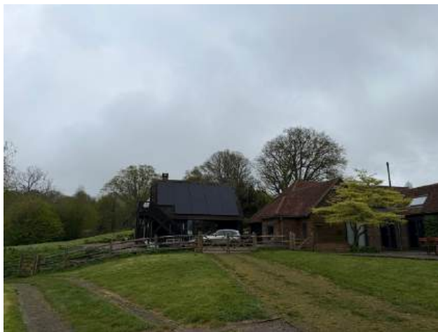
Plate 7 View showing solar panels in relationship with the ancillary structures.
