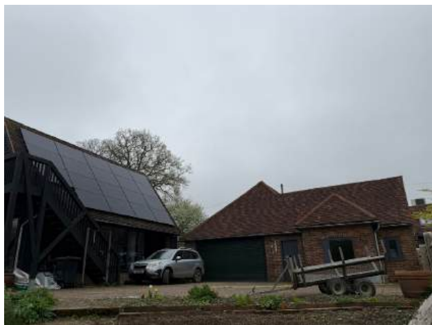
Plate 6 The solar panels are clearly visible in relation to the ancillary outbuildings which have been extensively altered and extended over time.
