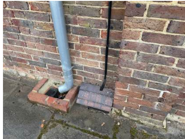
Plate 13 Connection of electricity cable into the ancillary structure.
