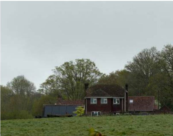
Plate 9 Showing how the solar panels blend in with the dark tones of the buildings within the site.
