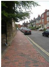
Red/multi brick pavers
