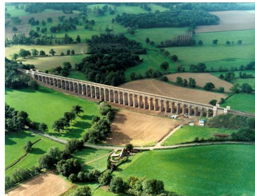
Ouse Valley Viaduct, 1841
