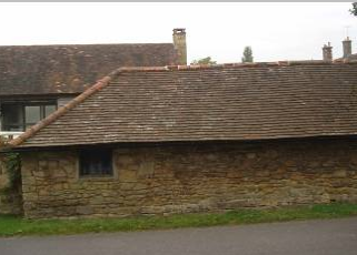
Stone farm out building
