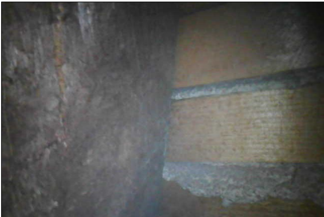
Appendix 2.16: Detail from inspection camera of timber stud and lath and plaster north wall in Room I-14 , (Observation 8) looking north
