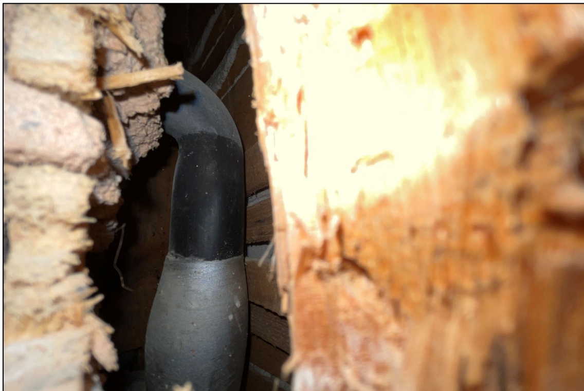
Appendix 2.18: Detail of lath and plaster east wall in Room I-14 , (Observation 9) looking north-east
