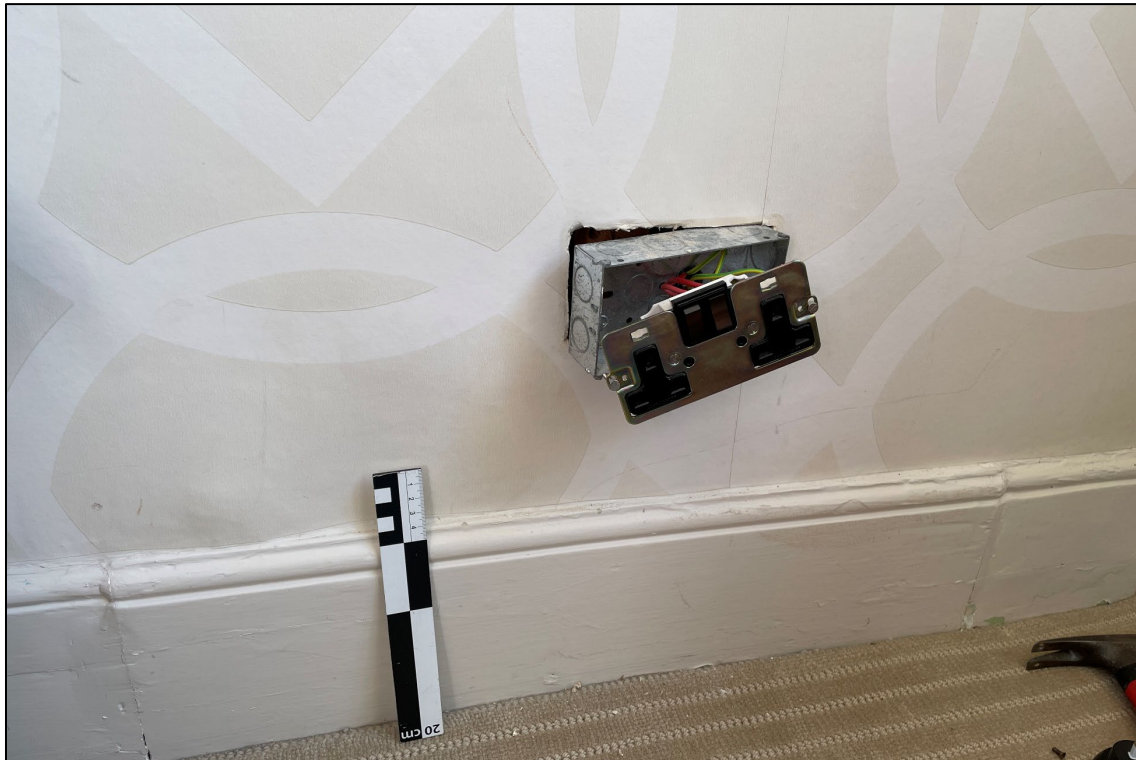
Appendix 2.17: Detail of disturbed skirting board on east wall in Room I-14 , (Observation 9) looking south-east (20cm Scale)
