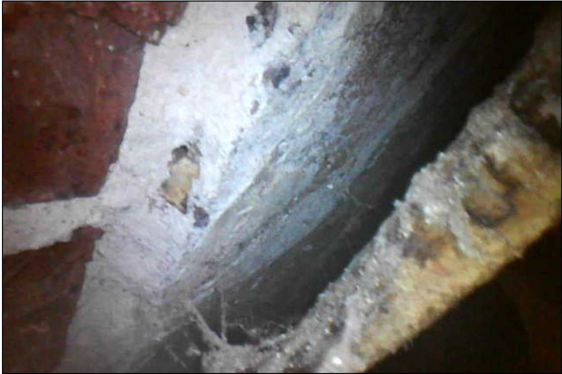
Appendix 2.11: Detail of lime plaster, Room 0-16 (Observation 3), looking north-east
