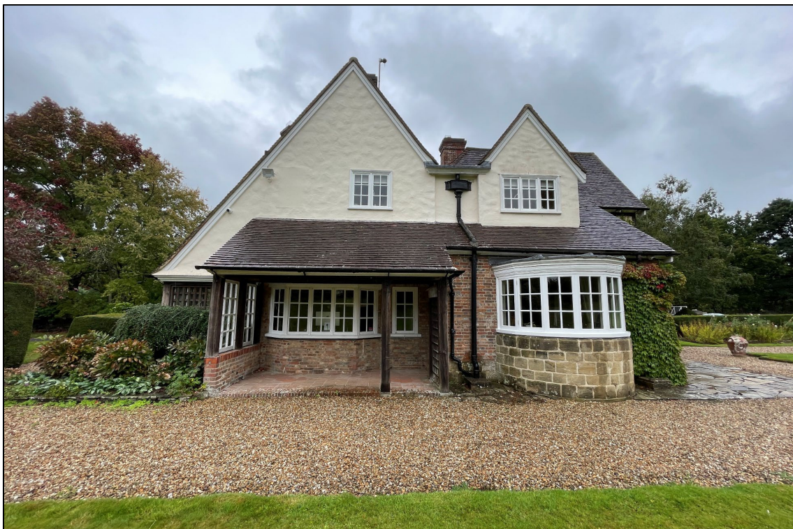
Appendix 2.2: General view of early-20 th century extension, looking east
