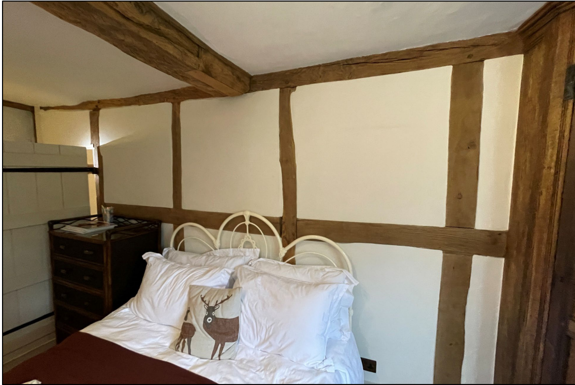
Appendix 2.7: General view of cross frame, Room 1-22 , looking west
