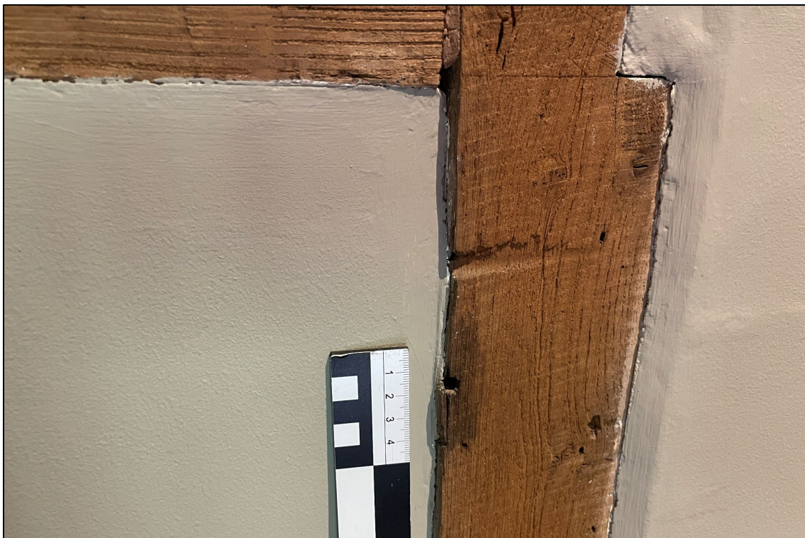
Appendix 2.4: Detail of reused timber in blocking, Room 0-11 , looking south (5cm Scale)
