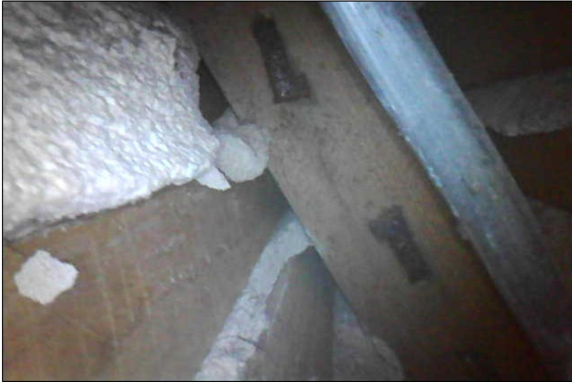
Appendix 2.15: Detail from inspection camera of lath and plaster south wall in Room I-15 , (Observation 7) looking east
