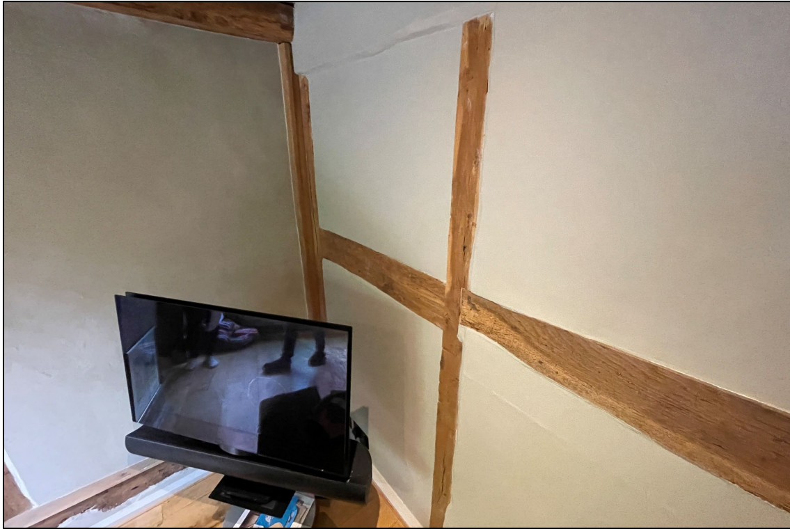
Appendix 2.3: General view of blocked door in Room 0-11 , looking south-east
