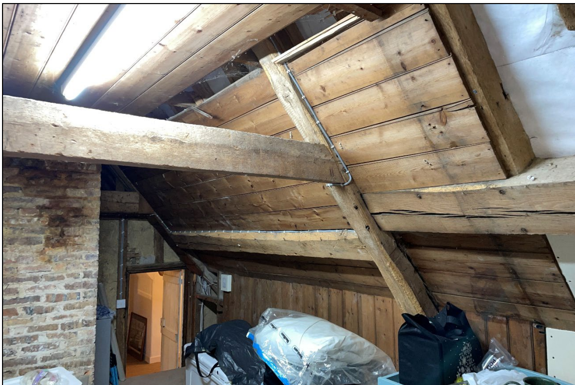
Appendix 2.8: General view of roof space, Room 2-05 , looking south-east
