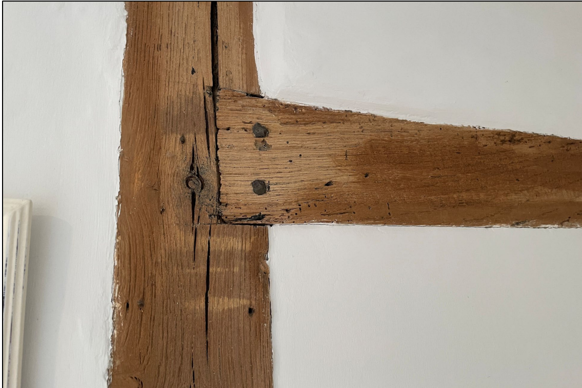
Appendix 2.5: Detail of infill to blocked door in Room 0-13 , looking north
