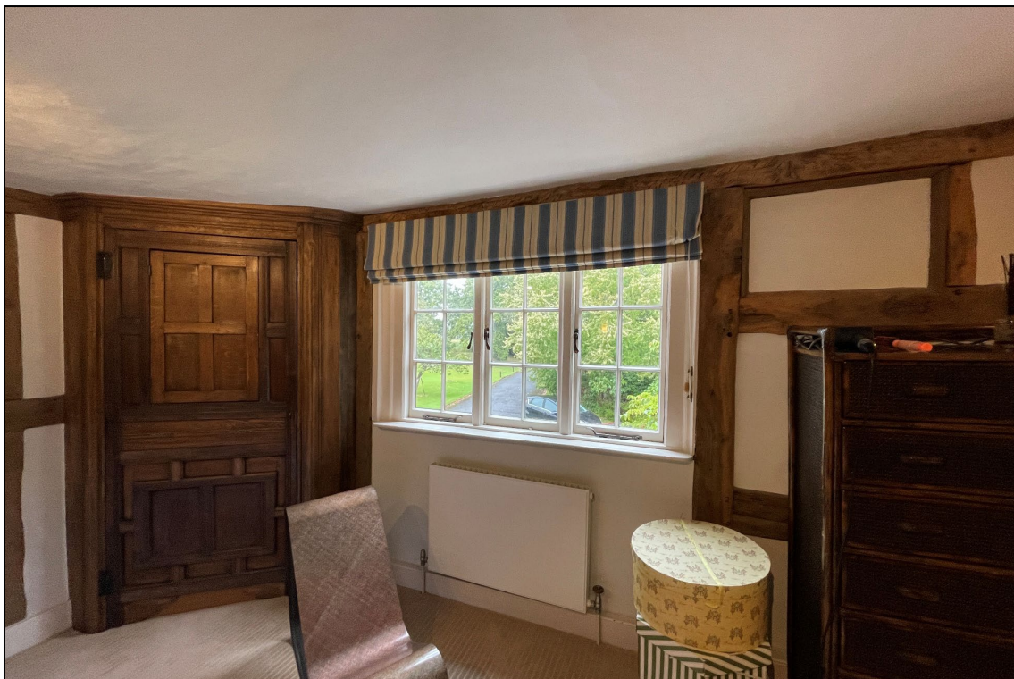
Appendix 2.6: General view of north wall and corner cupboard, Room 1-22 , looking north-west
