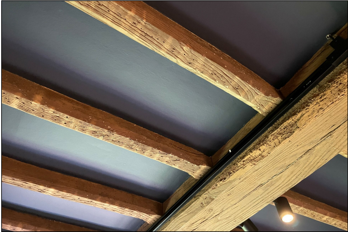
Appendix 2.13: Detail of chamfered ceiling beams, Room 0-09 , looking north-east
