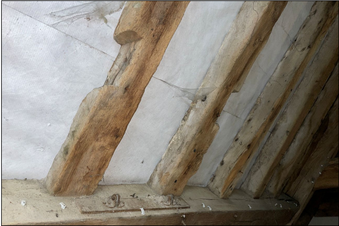
Appendix 2.9: Detail of reused common rafters, Room 2-05 , looking south-west
