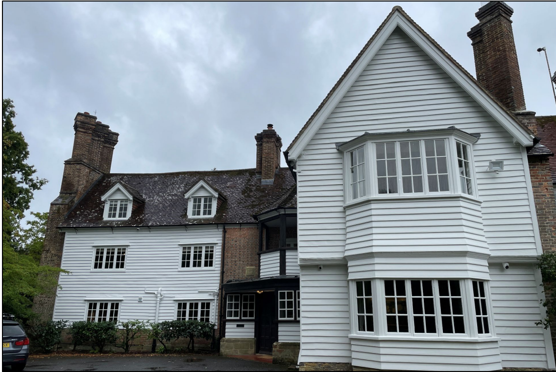
Appendix 2.1: General view of the house, looking south
