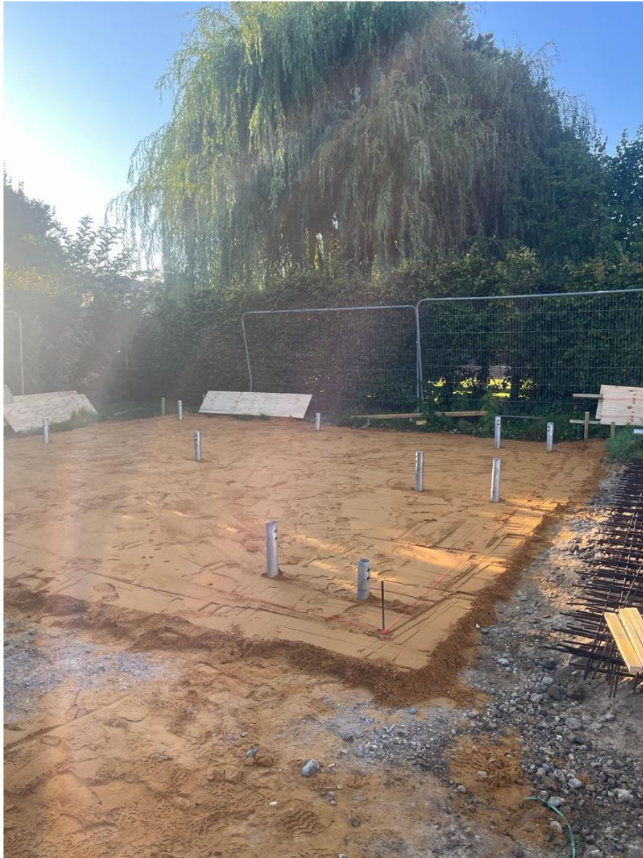
The screw piles all inserted and sticking though a layer of washed sand.
