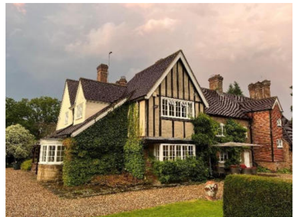
Plate 4. Southern elevation of Building B1 (from SW corner)
