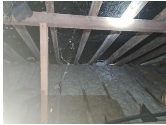
Plate 14. Internal aspect of Building B2's loft void
