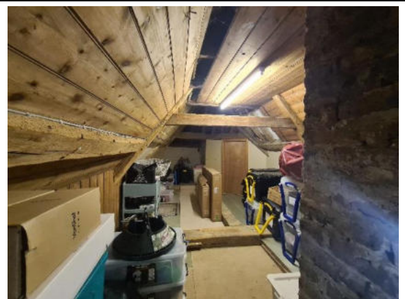
Plate 6. Internal aspect of Building B1's main loft void
