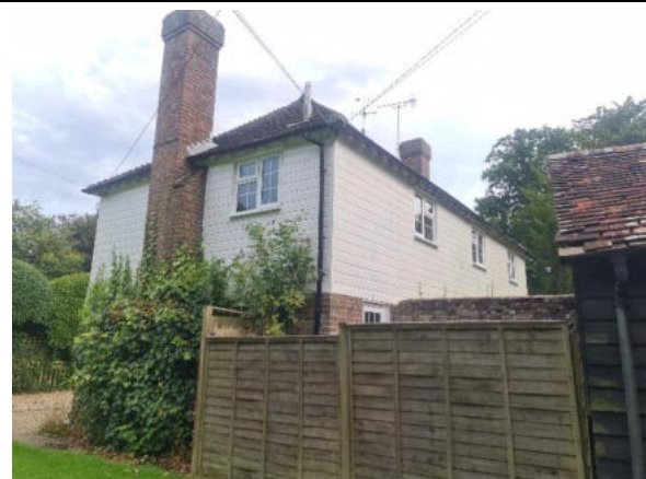
Plate 12. Northern elevation (left) and western elevation (right) from the northwestern corner of Building B2
