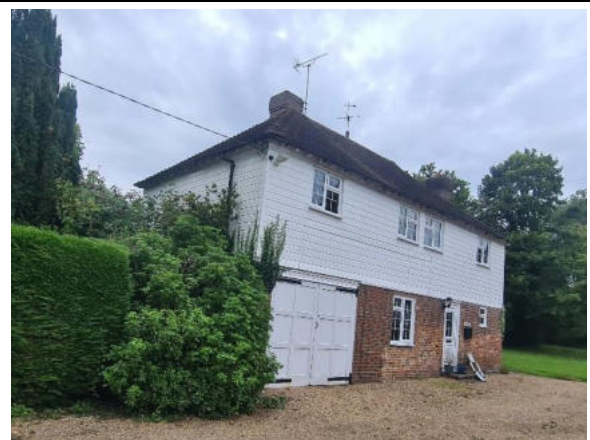
Plate 10. Southern elevation (left) and eastern elevation (right) from southeastern corner of Building B2
