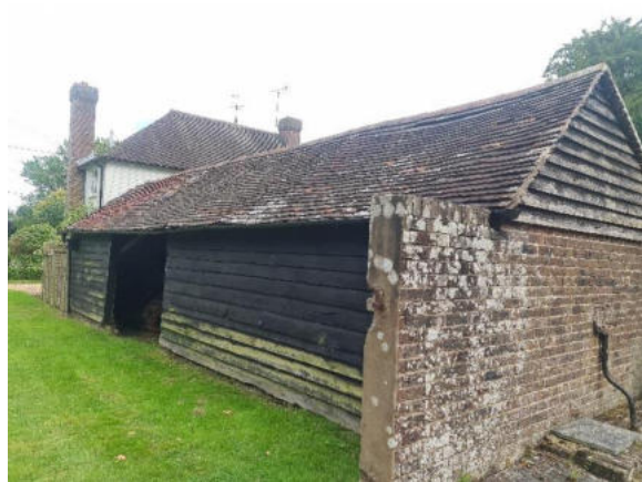
Plate 15. Outbuilding B3 – north-west aspect
