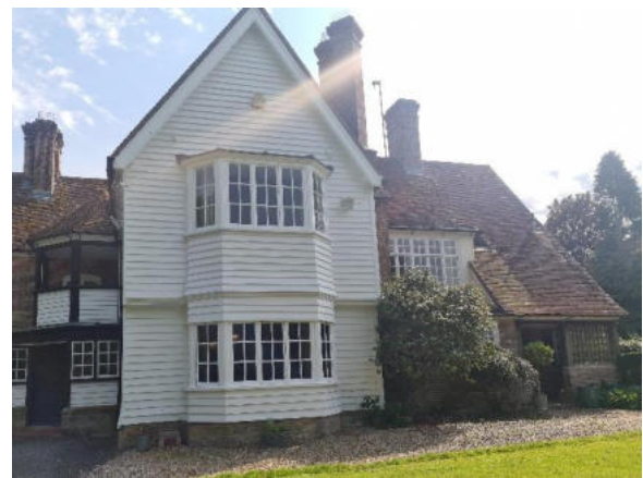
Plate 2. Northern elevation of Building B1 (NW section)
