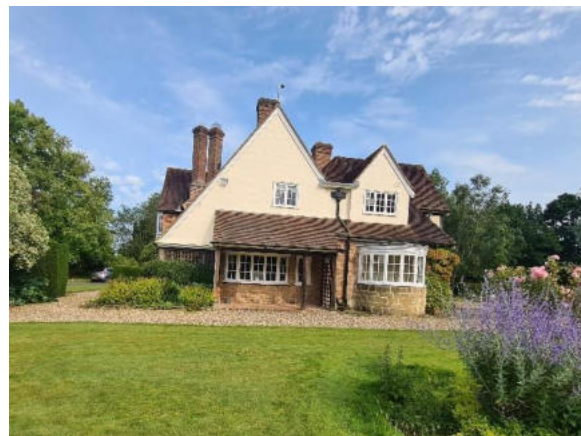
Plate 3. Western elevation of Building B1
