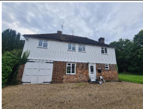
Plate 9. Eastern elevation of Building B2
