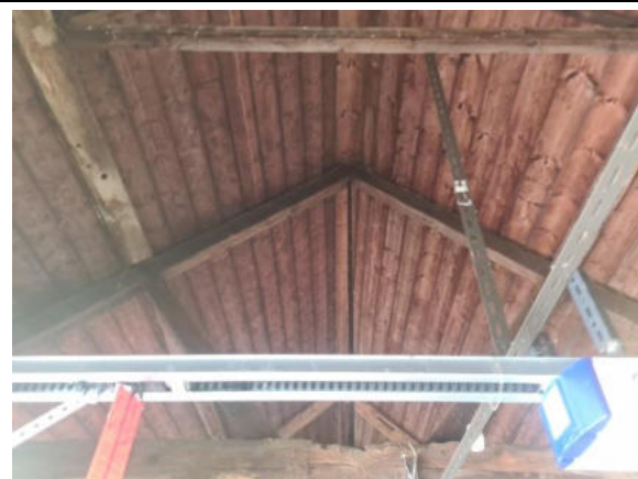
Plate 18. Internal view of B4
