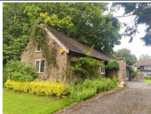
Plate 17. Barn B4 – south-west aspect
