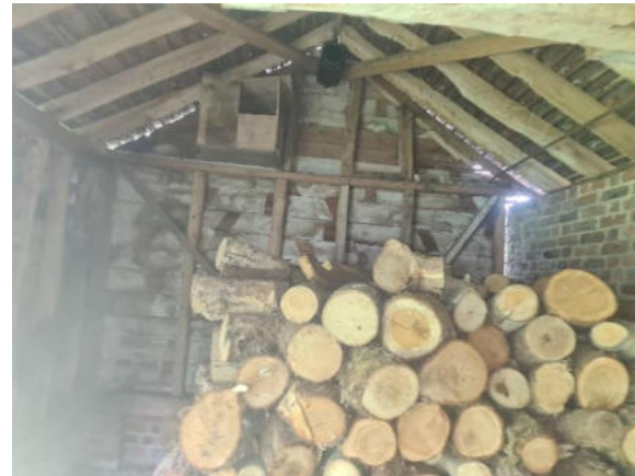
Plate 16. Internal view of B3
