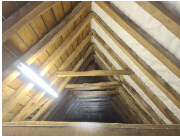
Plate 7. Timber frames in main loft void
