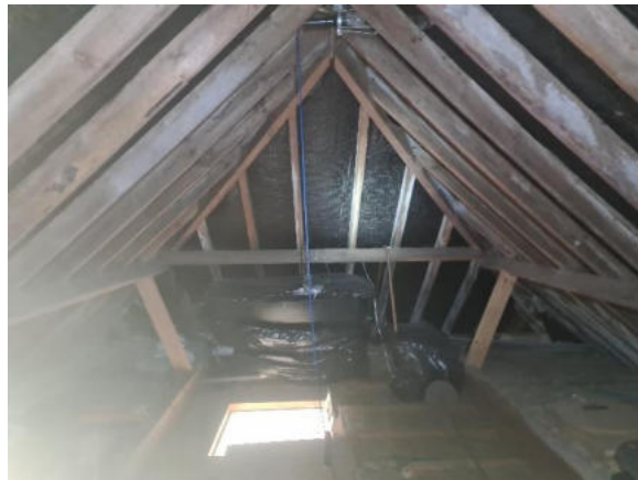
Plate 13. Internal aspect of Building B2's loft void
