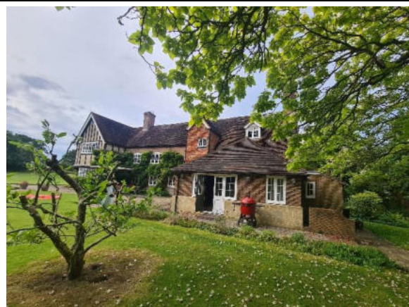
Plate 5. Southern elevation of Building B1 (from SE corner)
