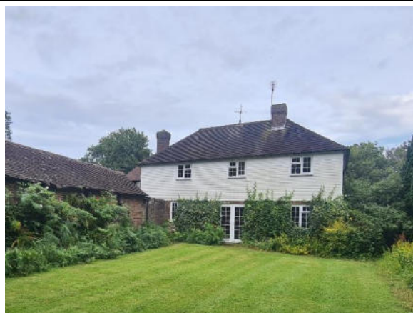
Plate 11. Western elevation of Building B2
