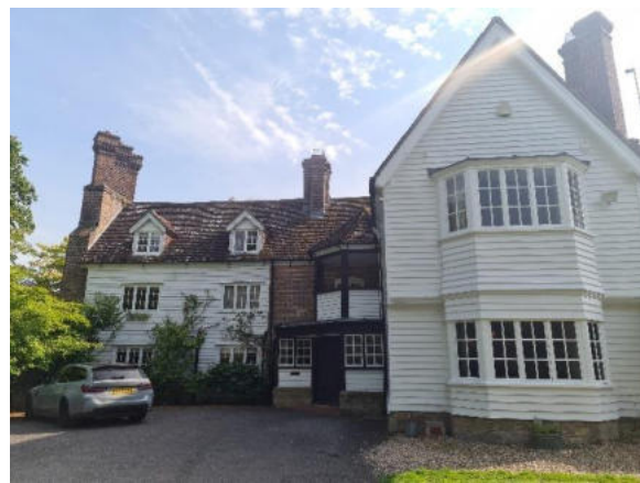
Plate 1. Northern elevation of Building B1 (NE section)
