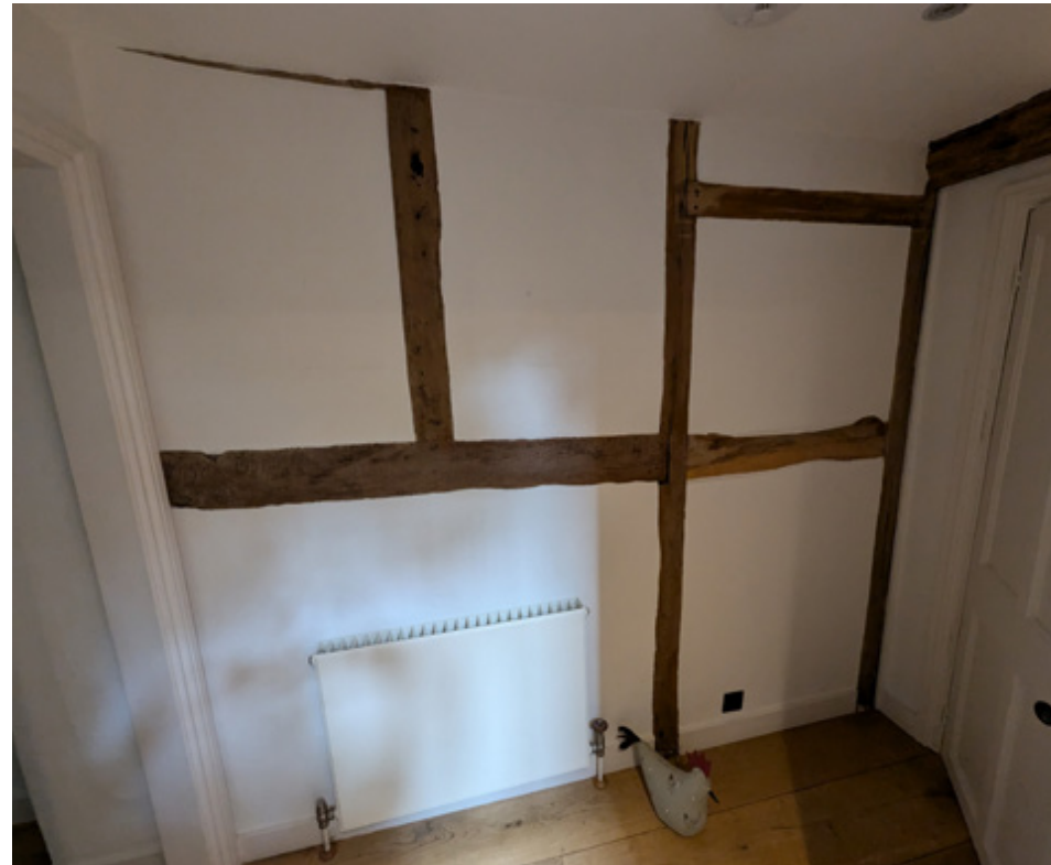
05. Walls in Snug, west of existing kitchen
