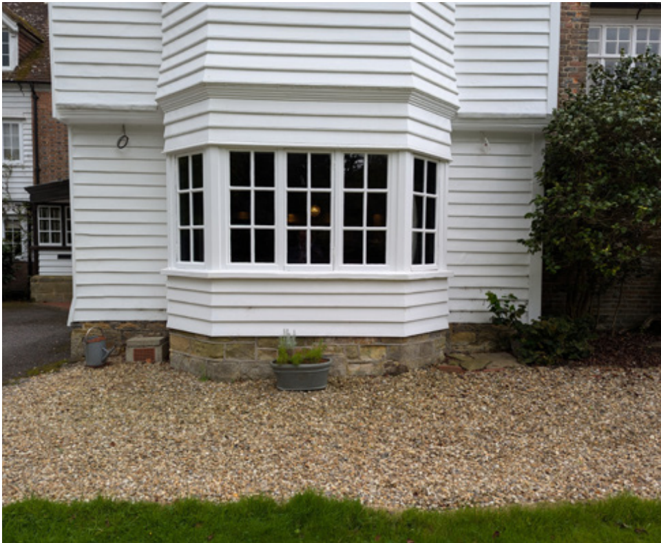
08. Bay window to north wing
