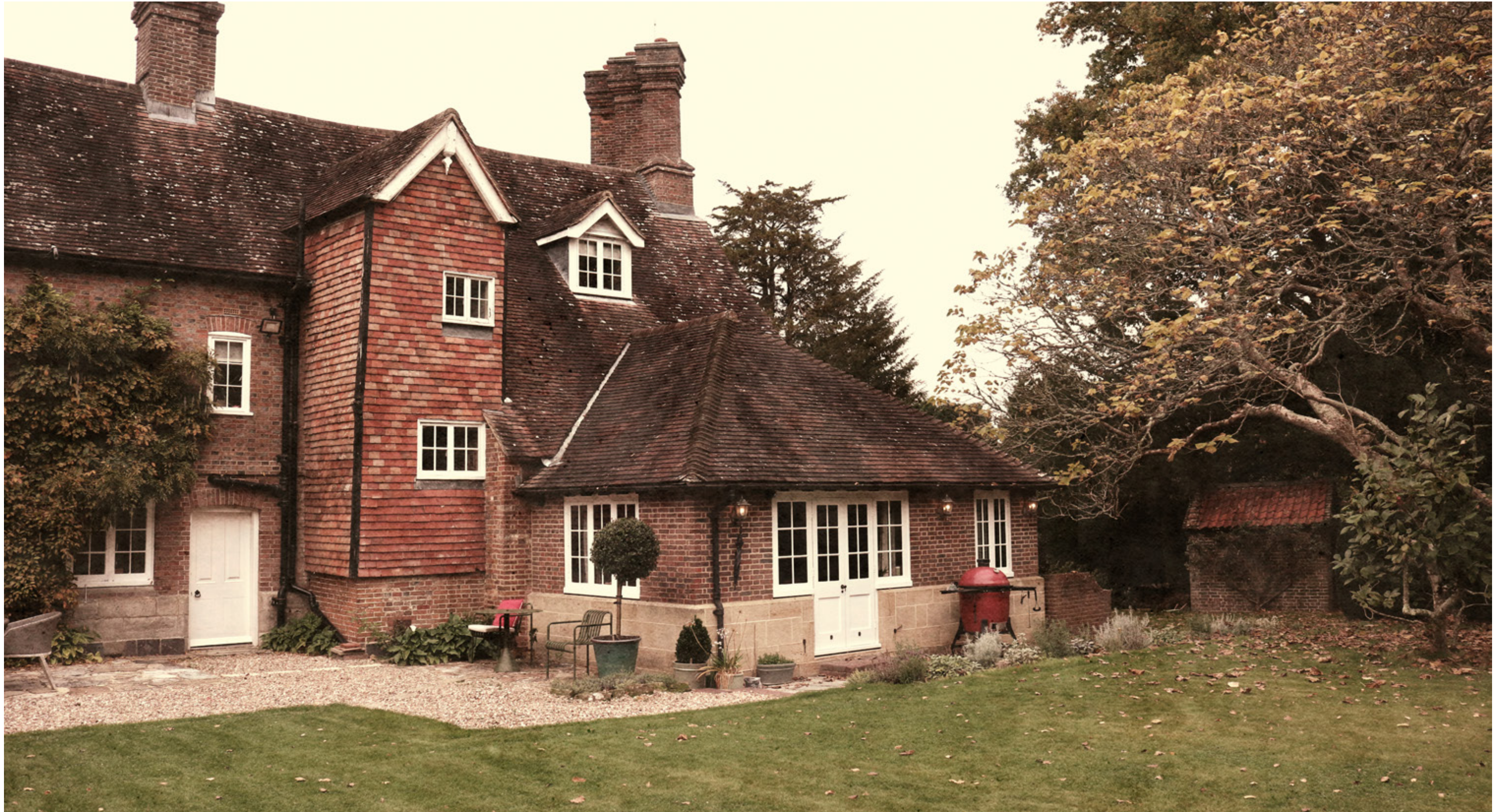
Existing view of east end of south elevation
