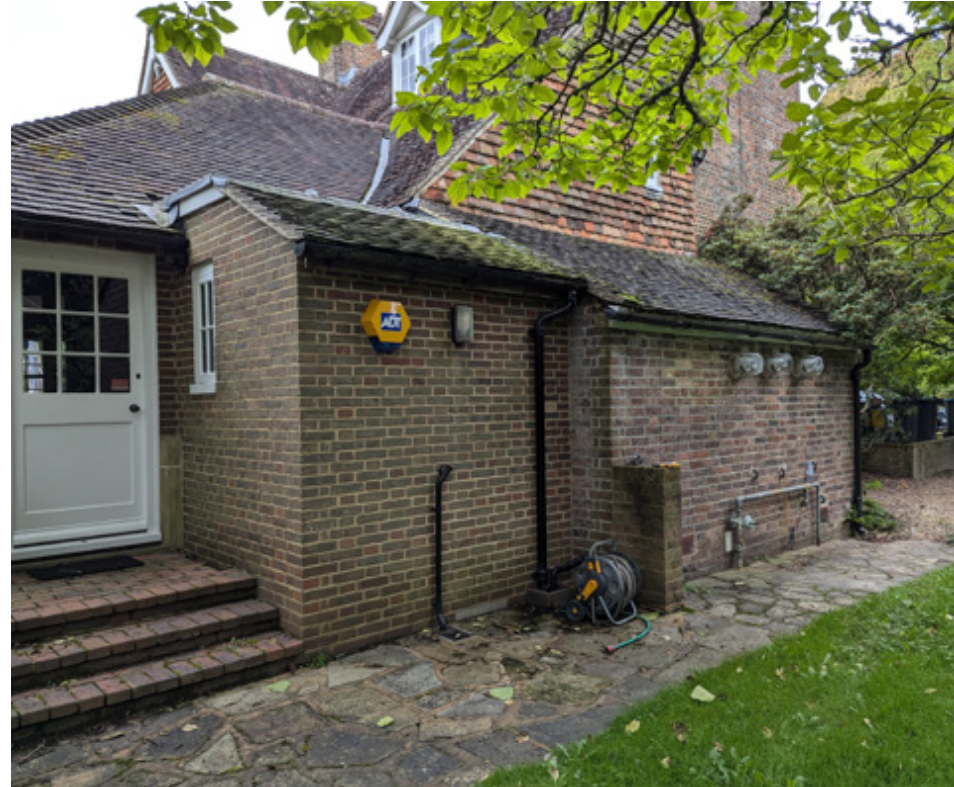
02. Lean-to additions to east elevation
