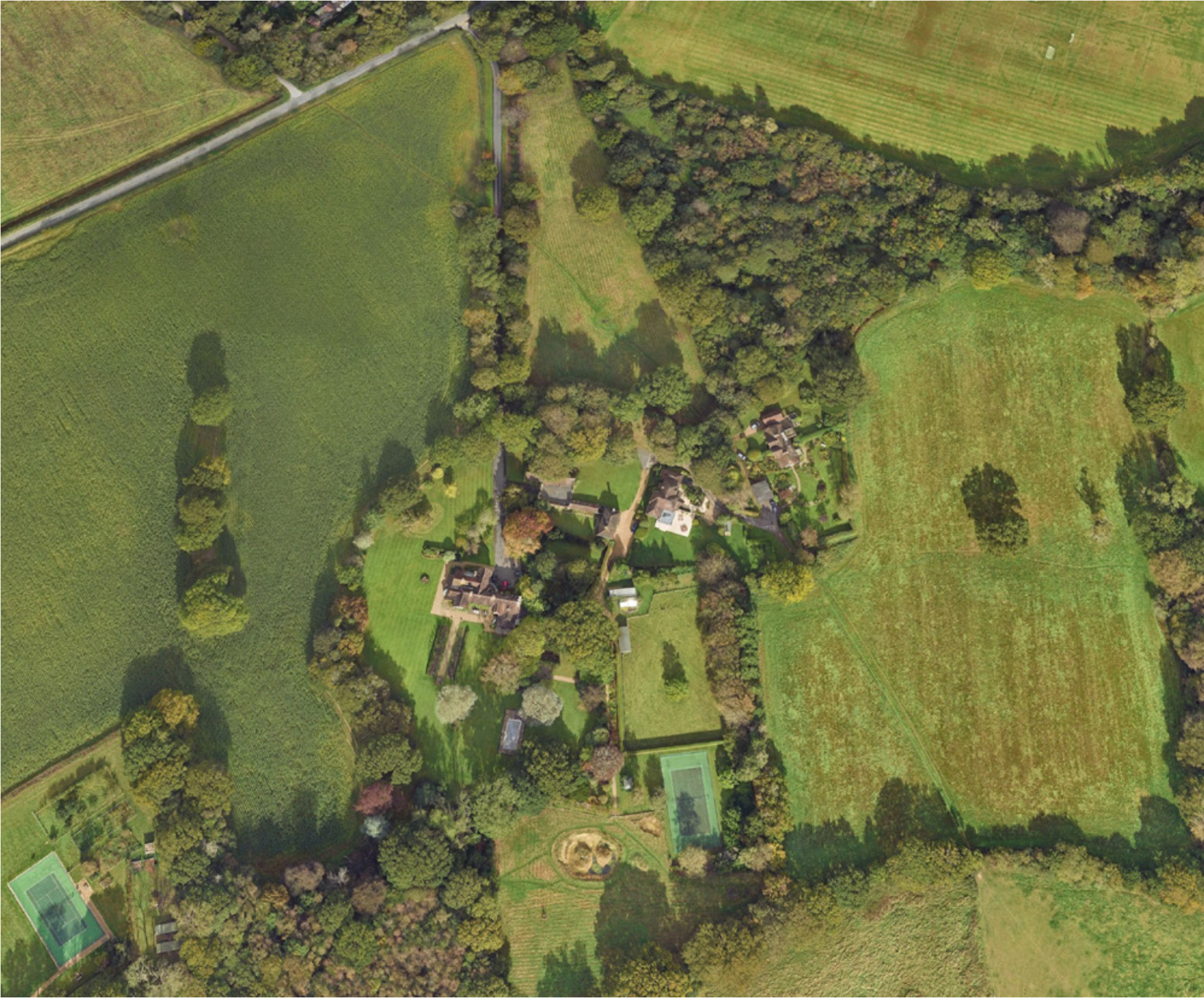
Aerial view of Nether Walstead and neighbouring cottages.
