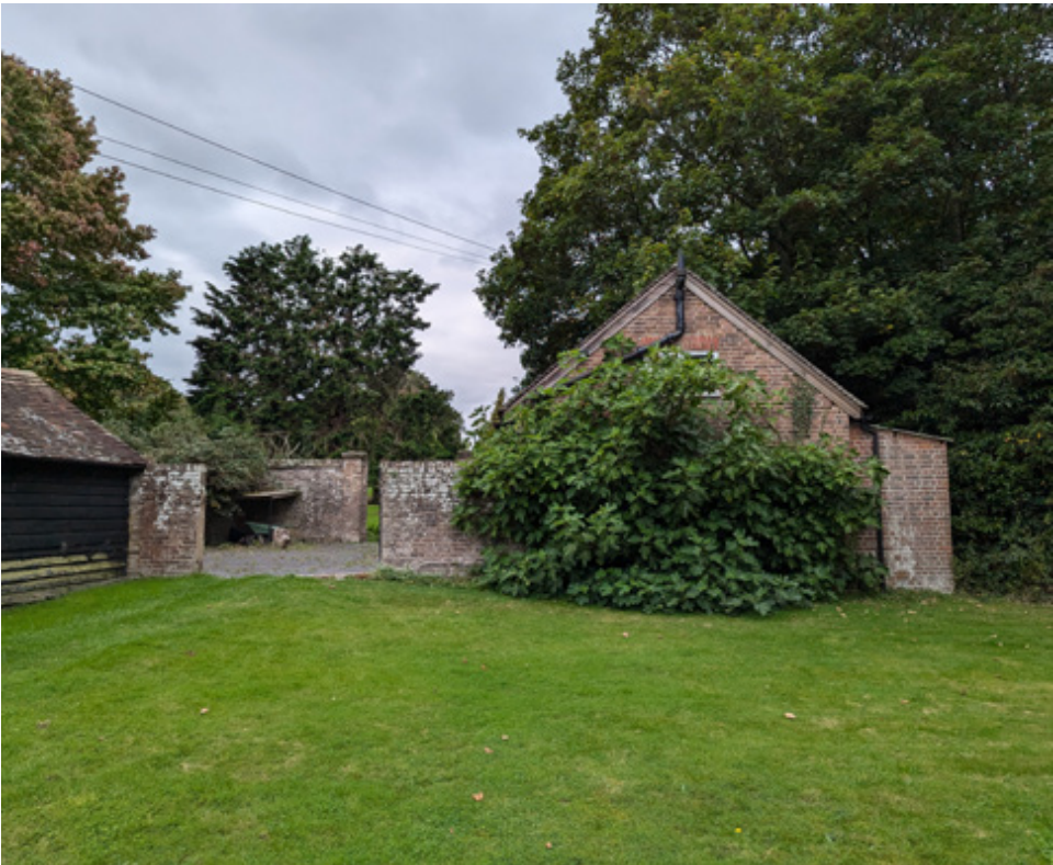
East side of garage and courtyard
