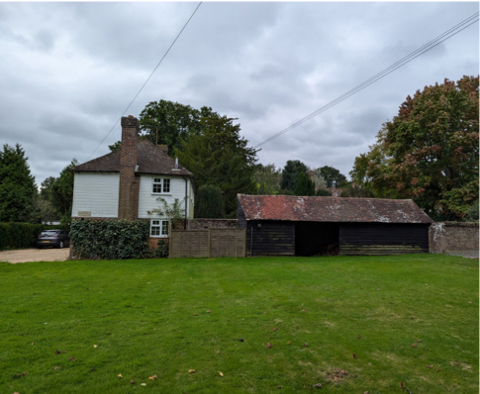
North side of Coach House and Wood Store
