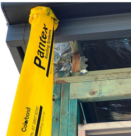
Example of temporary rwp connection
