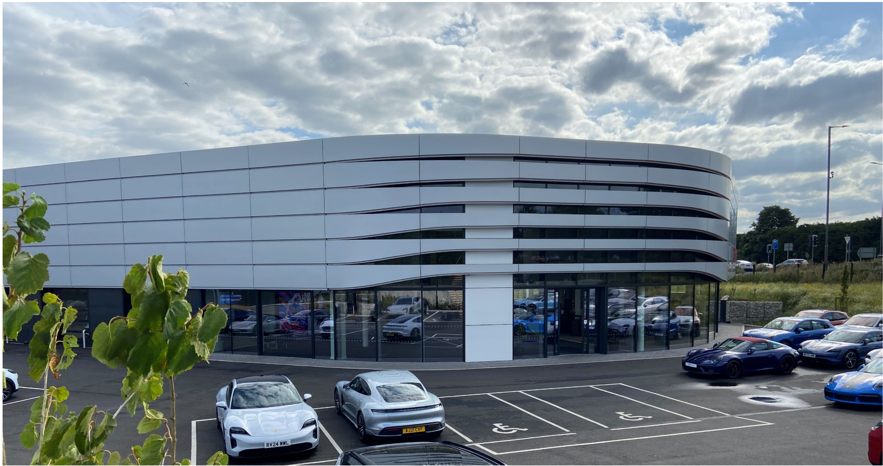
Alucabond rainscreen cladding in RAL 9006 Silver
