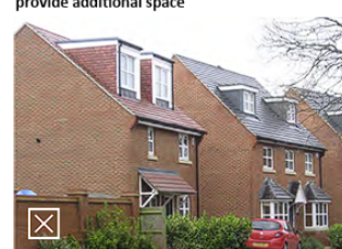
The dormers in the foreground were added and are too big and top heavy; the dormers in the background are by contrast appropriately sized
