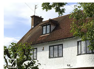
Dormers successfully integrated into the roof to provide additional space
