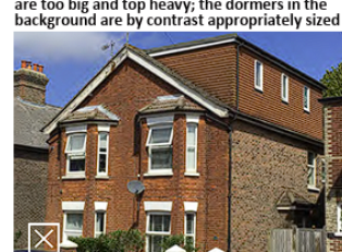
This over-sized dormer undermines the shape and symmetry of this gable frontage.
