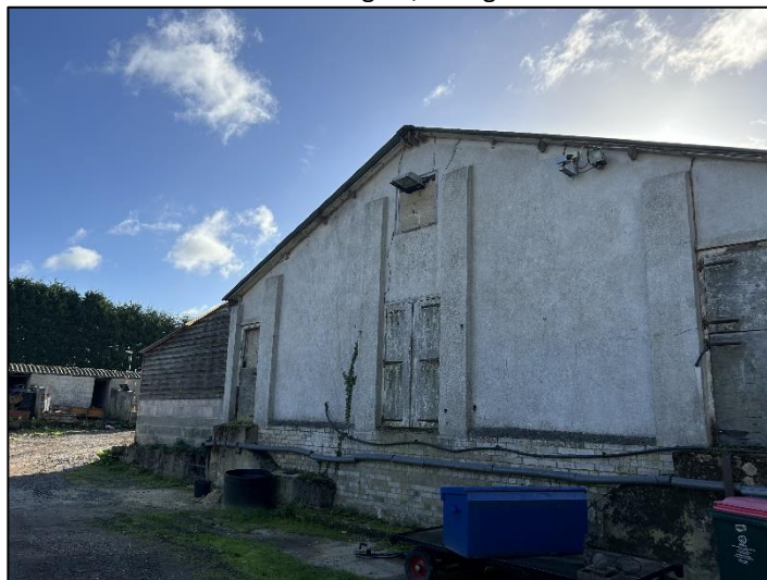
Photo 4.4: Building B1, facing south-east.
