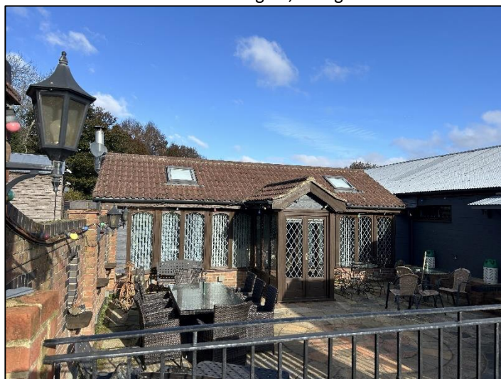
Photo 4.6: Building B1, facing north.
