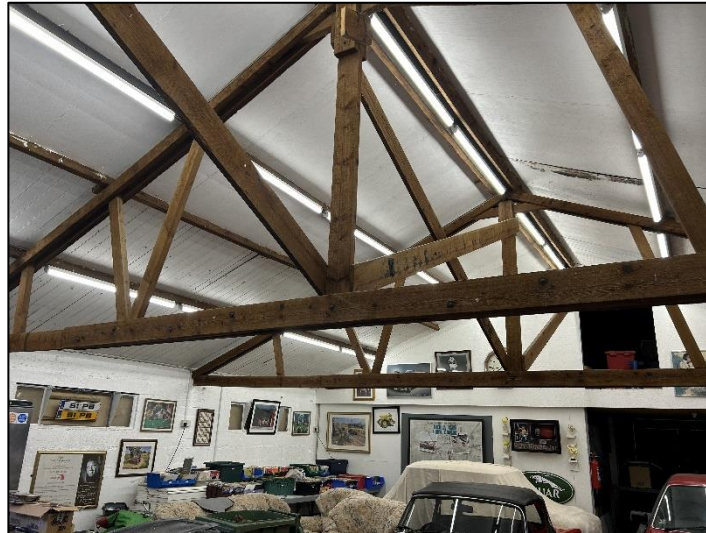
Photo 4.7: Building B1, internal area of the northern section of the building.
