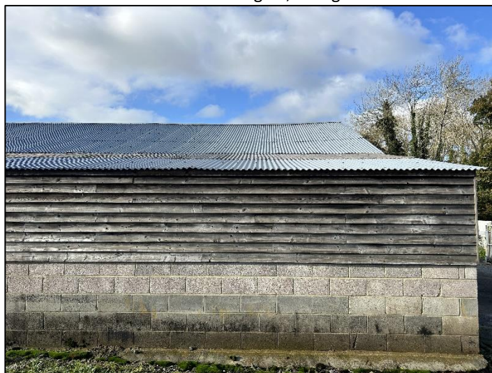
Photo 4.5: Building B1, facing west.
