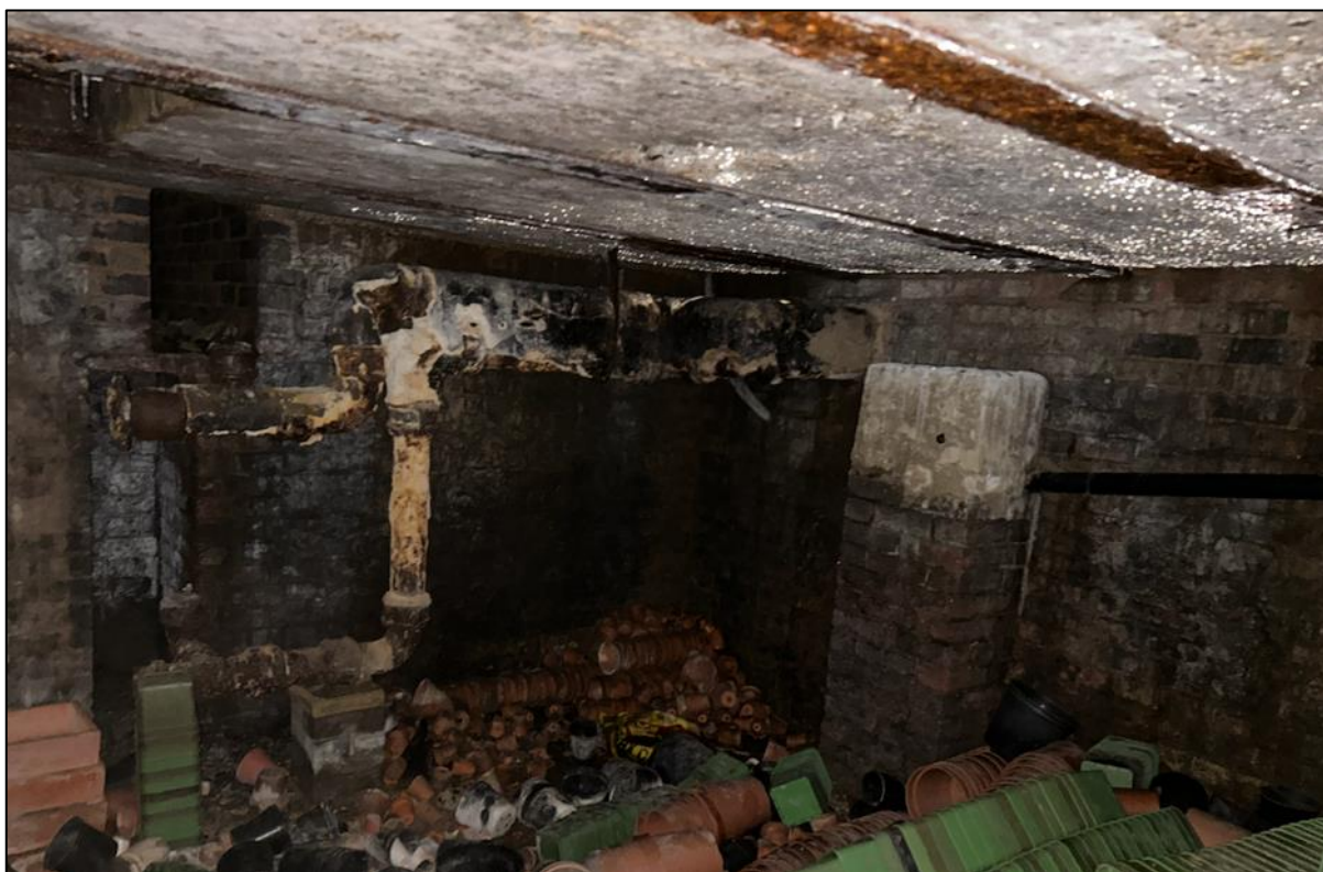
Photograph 4. An underground area understood to have formerly been used for heating a greenhouse.
