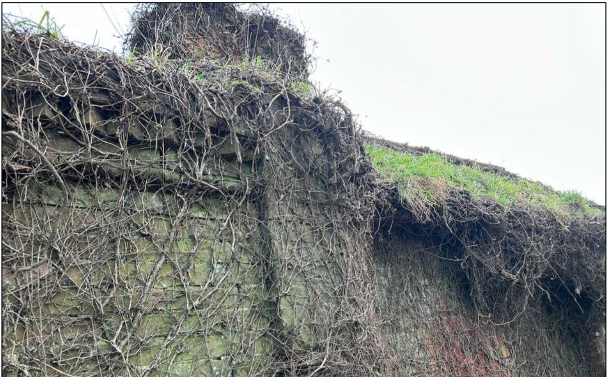
Photograph 2. A restricted view of the western face of the shed, which sits directly adjacent to the B2028
