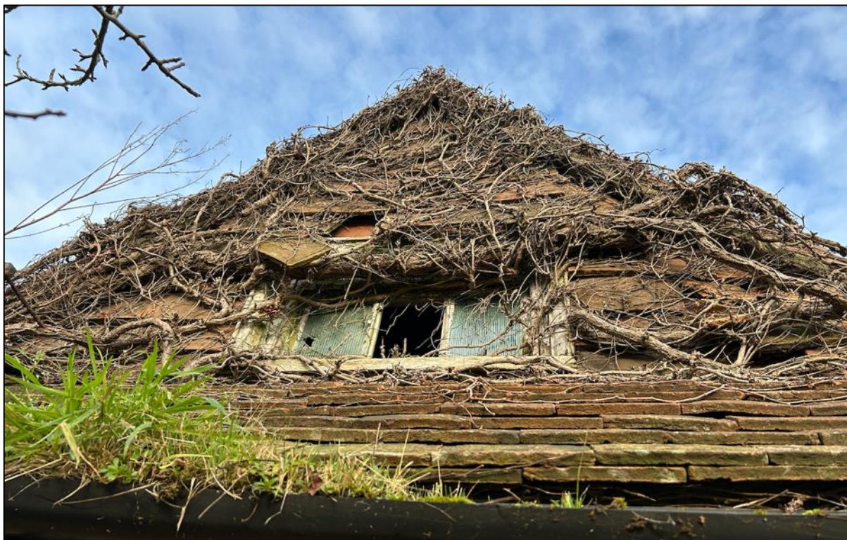
Photograph 3. The southern face of the building, where there are some large tile gaps there were closely inspected from a ladder. No evidence of use by bats was found.
