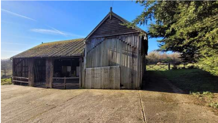
Existing East Elevation of Barn
