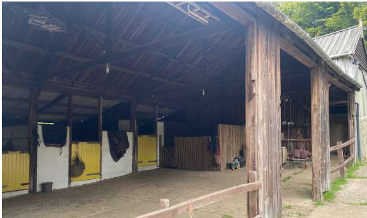
Interior of Existing Barn
