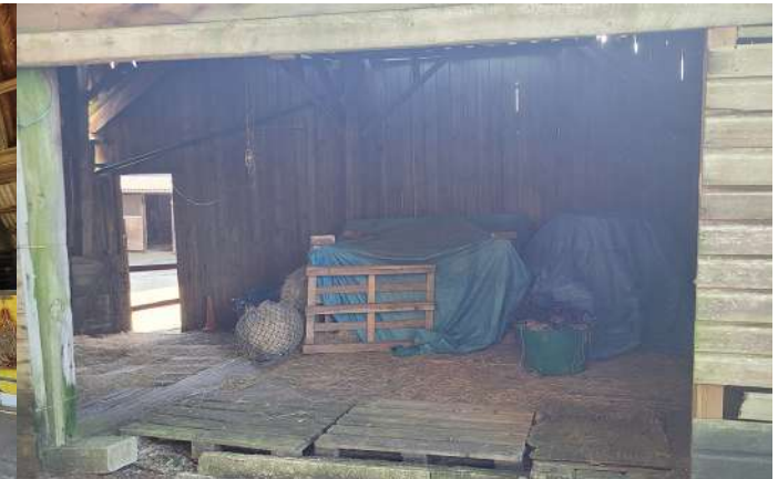
Interior of Existing Barn
