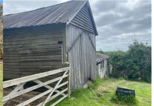
Existing West and part of North Elevation of Barn
