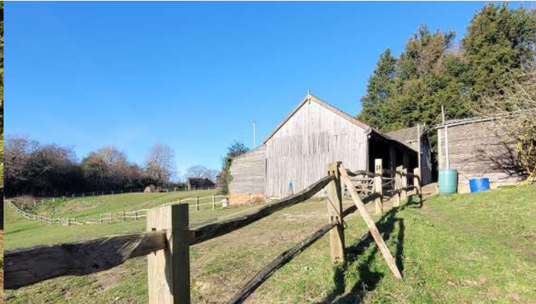
Existing South Elevation of Barn
