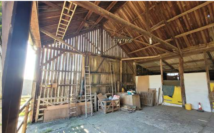
Interior of Existing Barn
