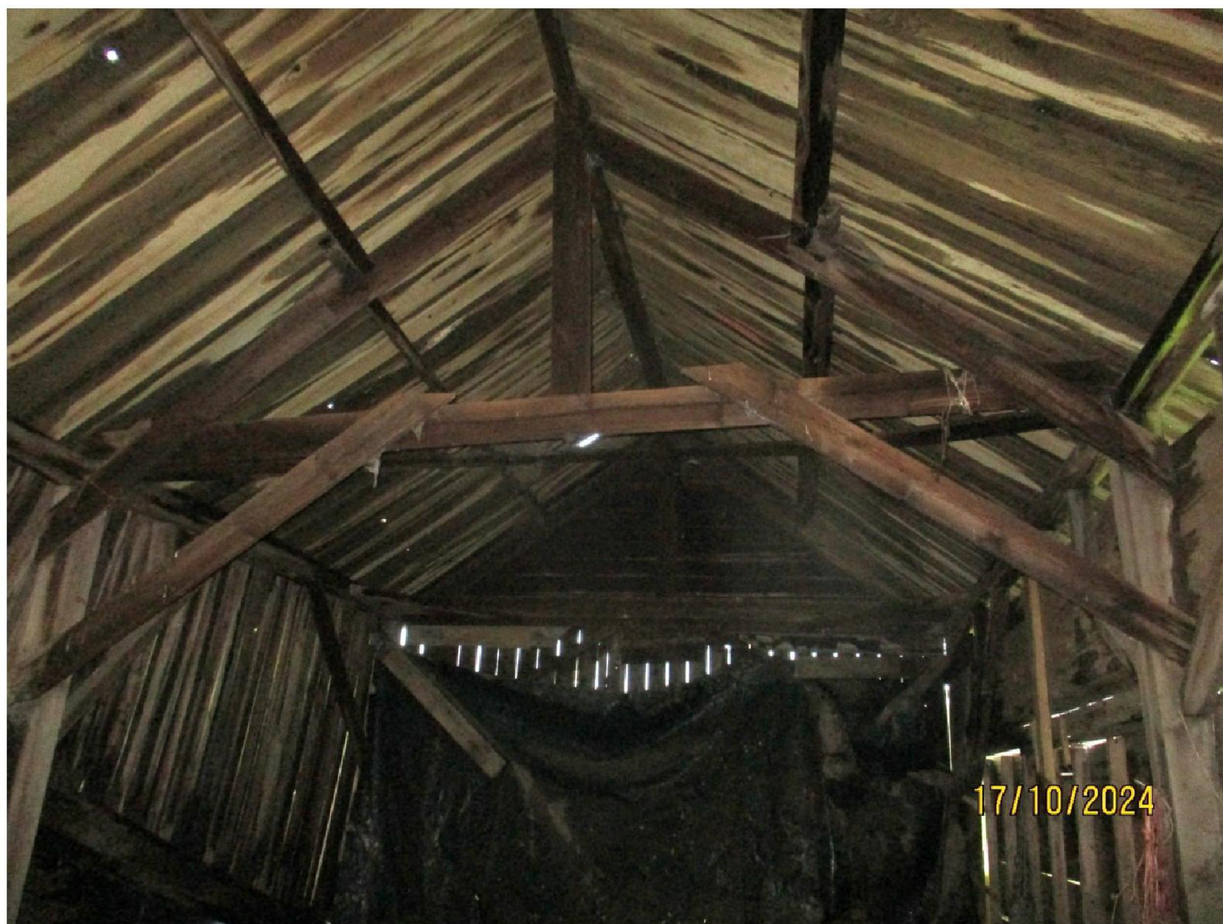
PHOTO #7– Internal view of Barn.
