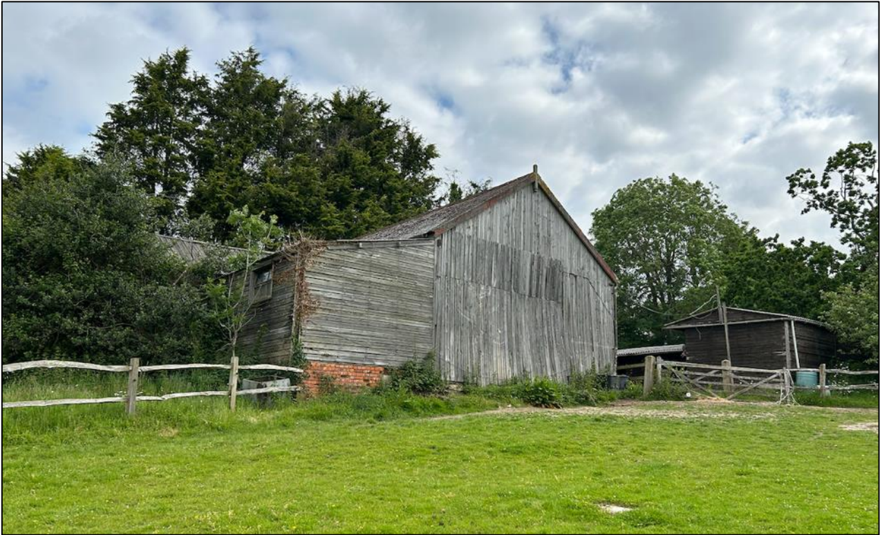
Photograph 4. The southern face of the large barn, with single-skin timber cladding on the gable end wall.
