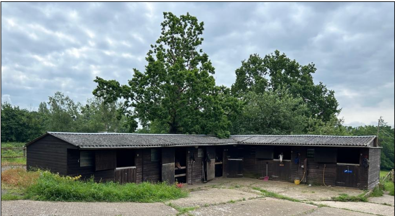
Photograph 5: View of the north-west aspect of the stables building, which are to be retained.
