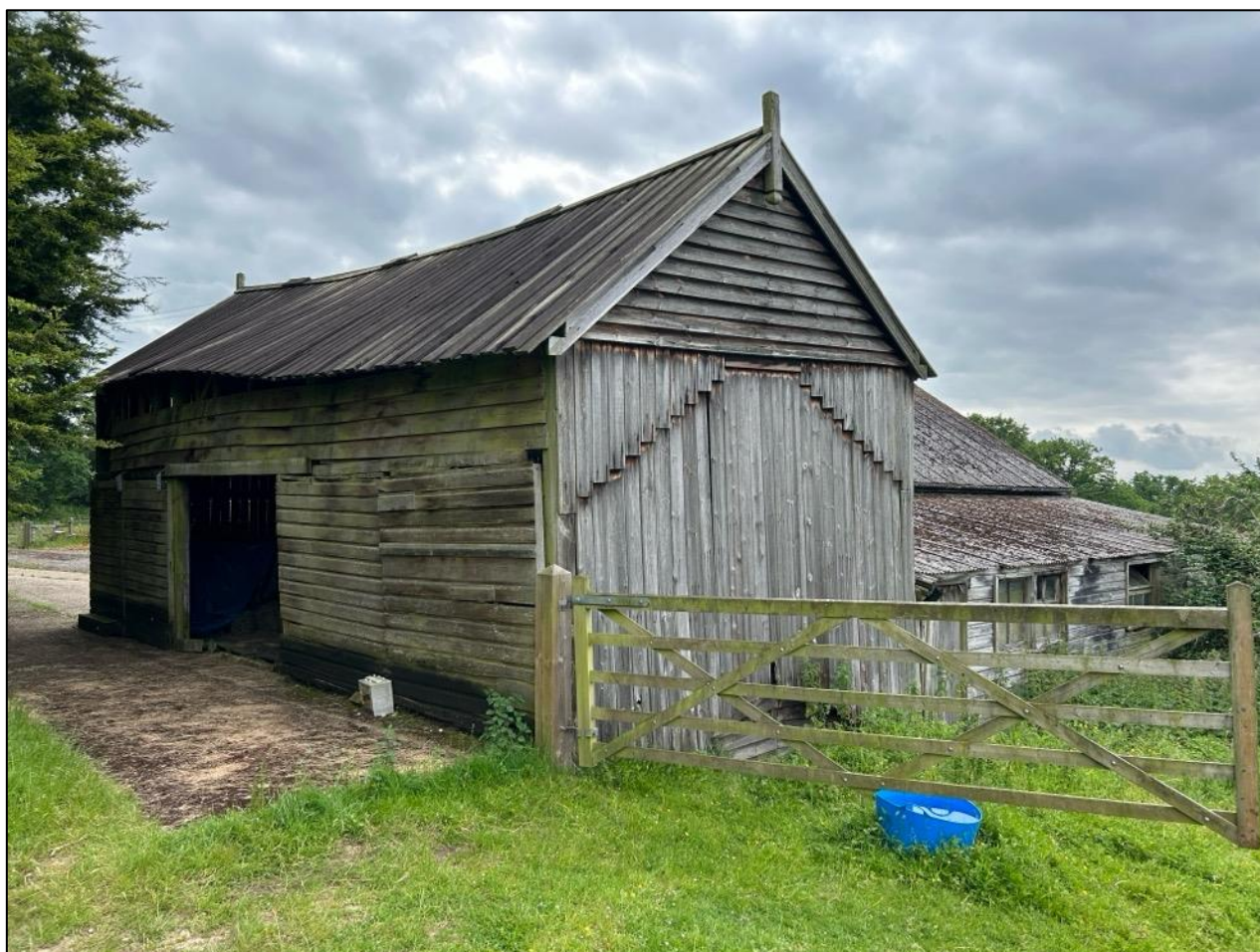
Photograph 3. A view of the northern and western aspects of the small barn which will be converted in the new development.
