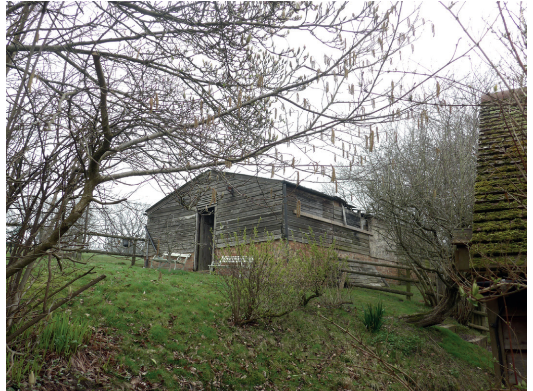
3. View of existing outbuilding
