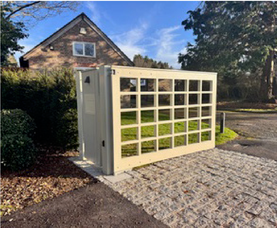
Gate 3 as installed
