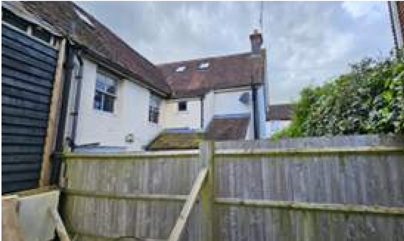
Former Rear and side of Somners with no outlook
