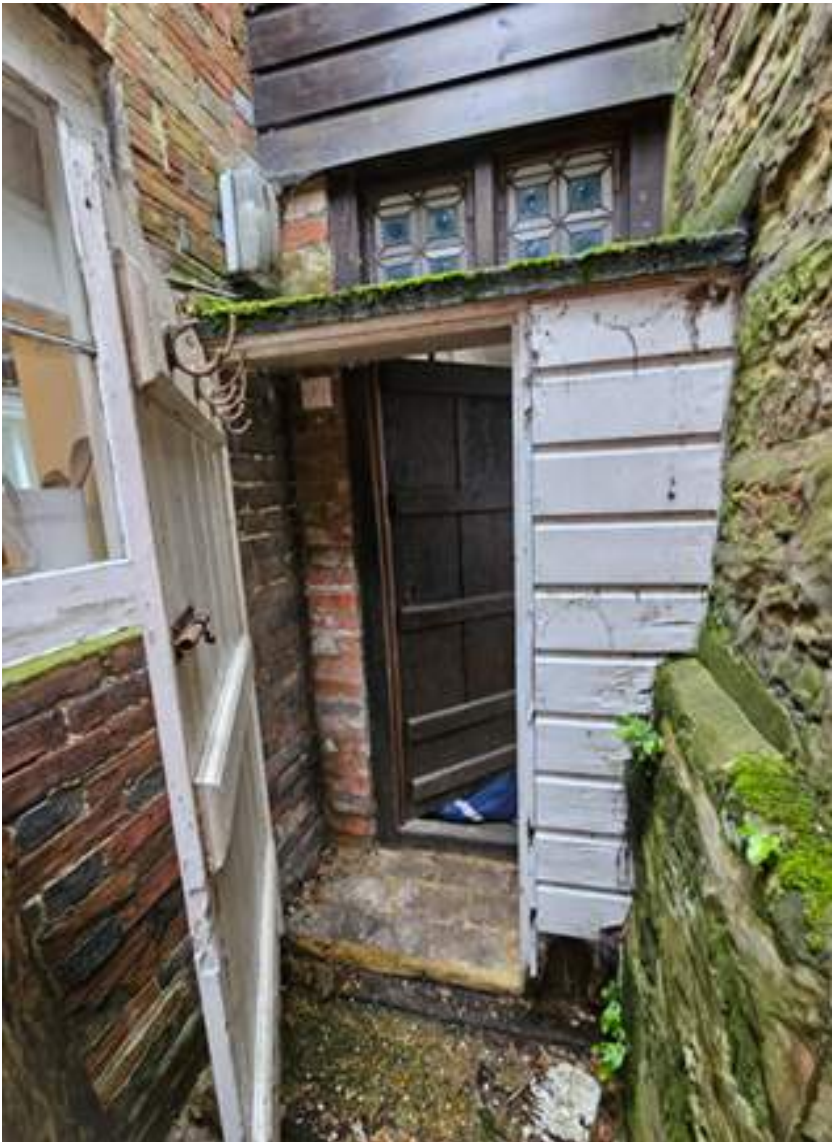
Modern wall and door to be removed.
