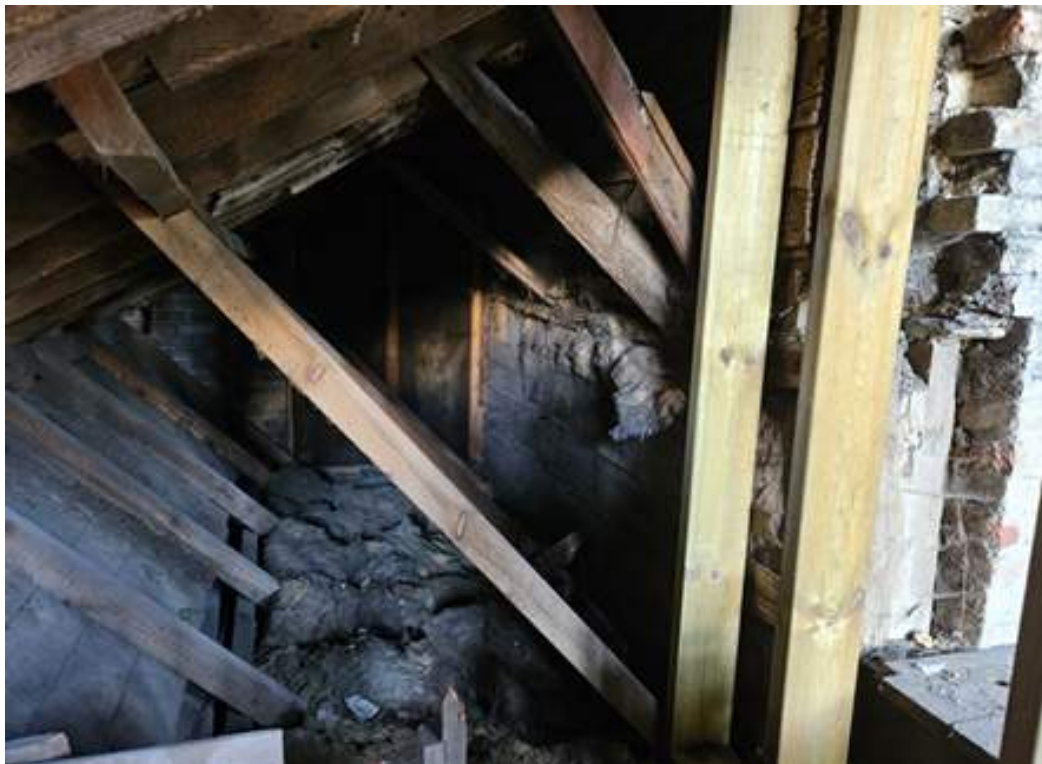
Images of the old roof to rear of The Friary. The later roof forming the catslide can be seen over, and boarding to the side of Somners revealed.
