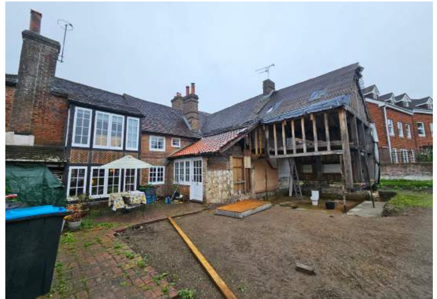
Picture showing former Dumbrells prior to demolition
