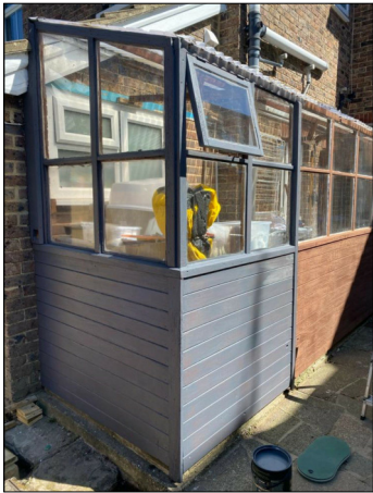
PRE EXIXTING LEANTO 2017 TO 2024
