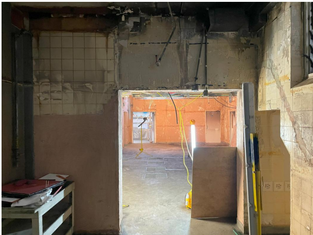
Internal view of Kitchen-Bakery
