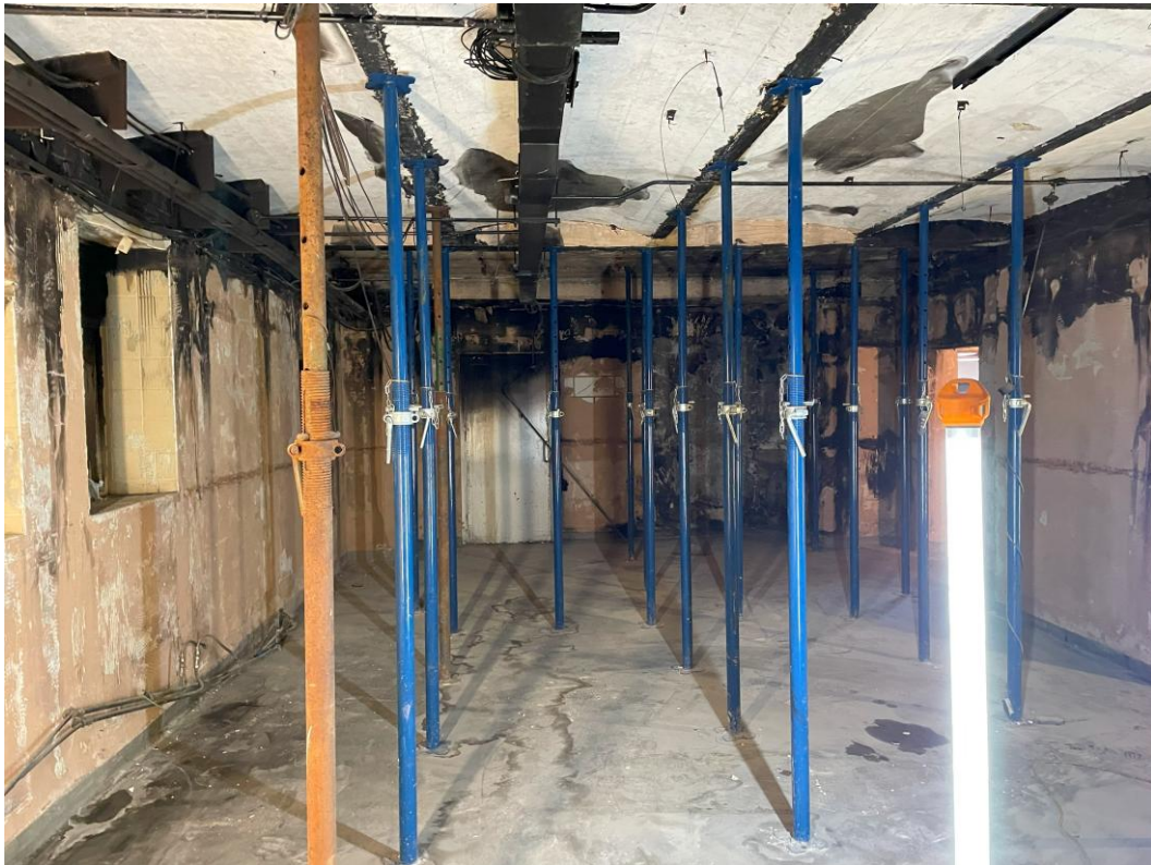
Internal view of kitchen-prep
