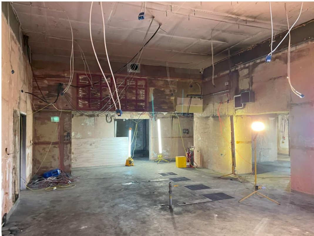
Internal view of kitchen-prep
