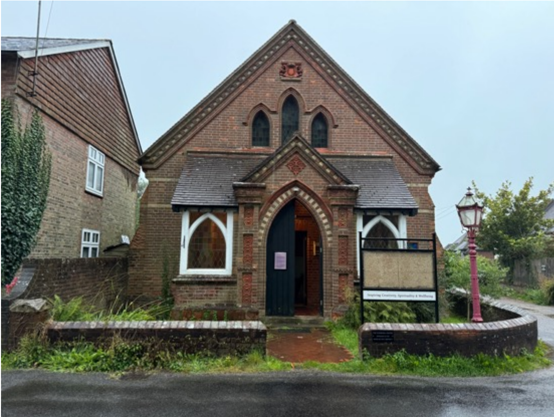
Photograph 1: Front (north) aspect, looking south
