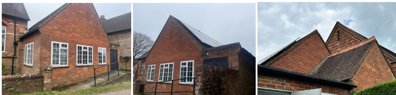
Figure 17: Series of more modern extensions to the south of the hall building.
