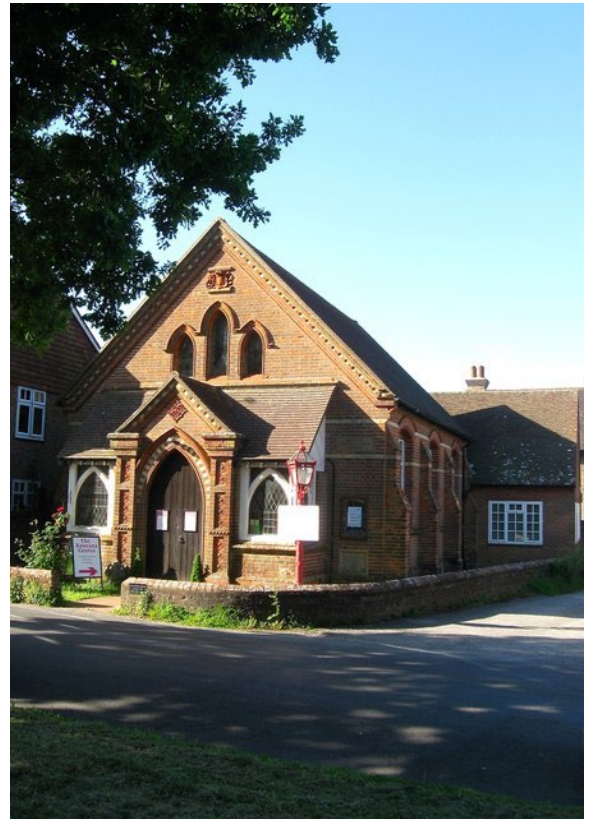
Figure 12: Former Congregational Church building used as a spiritual and therapy centre 2015.
