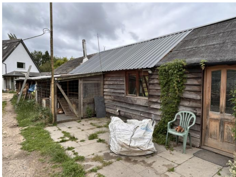
View of front of Dwelling 2 (to be demolished and replaced with extended dwelling 1)
