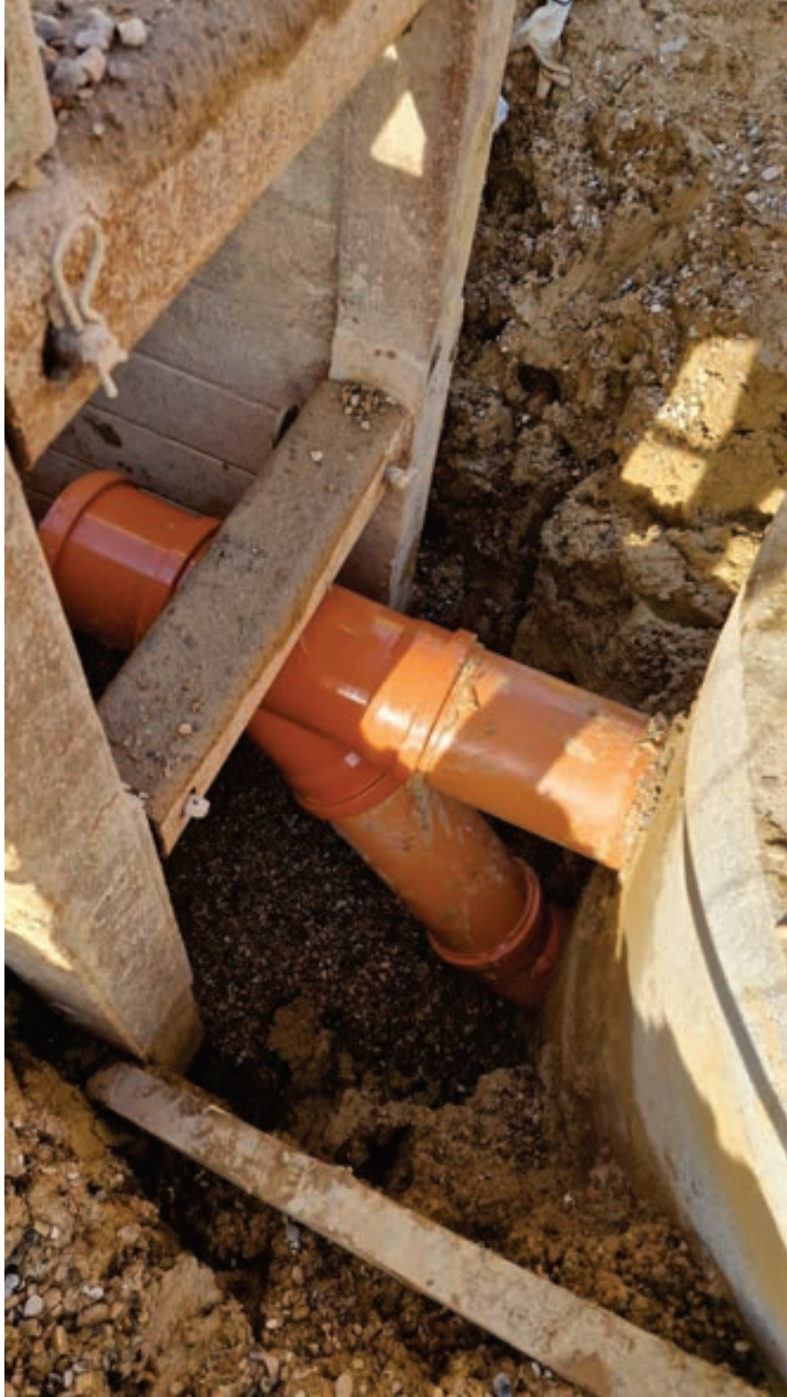
Photo 24 – Back drop to manhole S24
