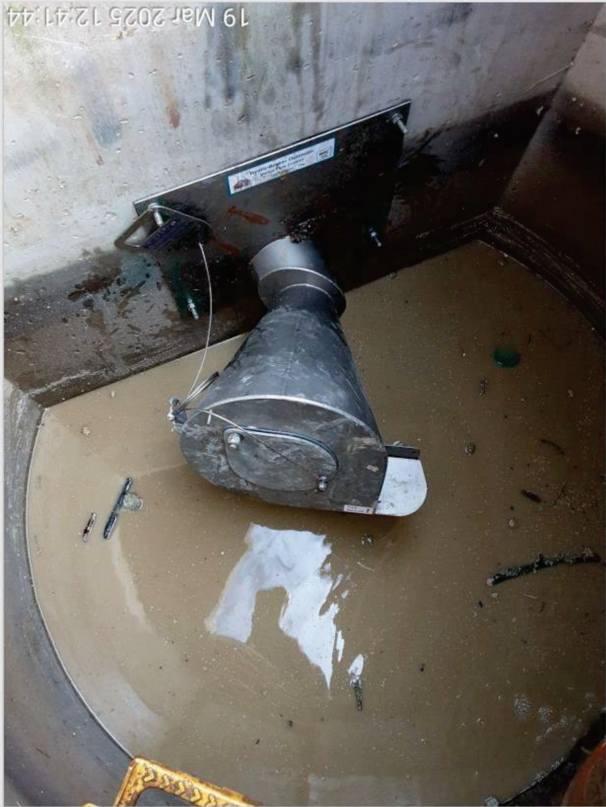
Photo 10 – Hydro-brake installed
