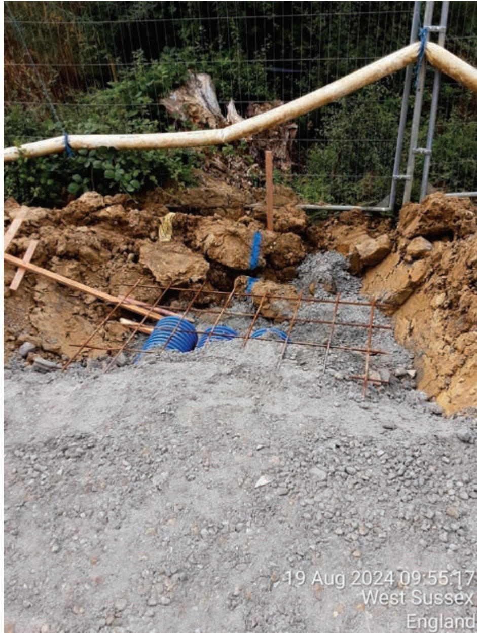
Photo 21 – Culvert C installation
