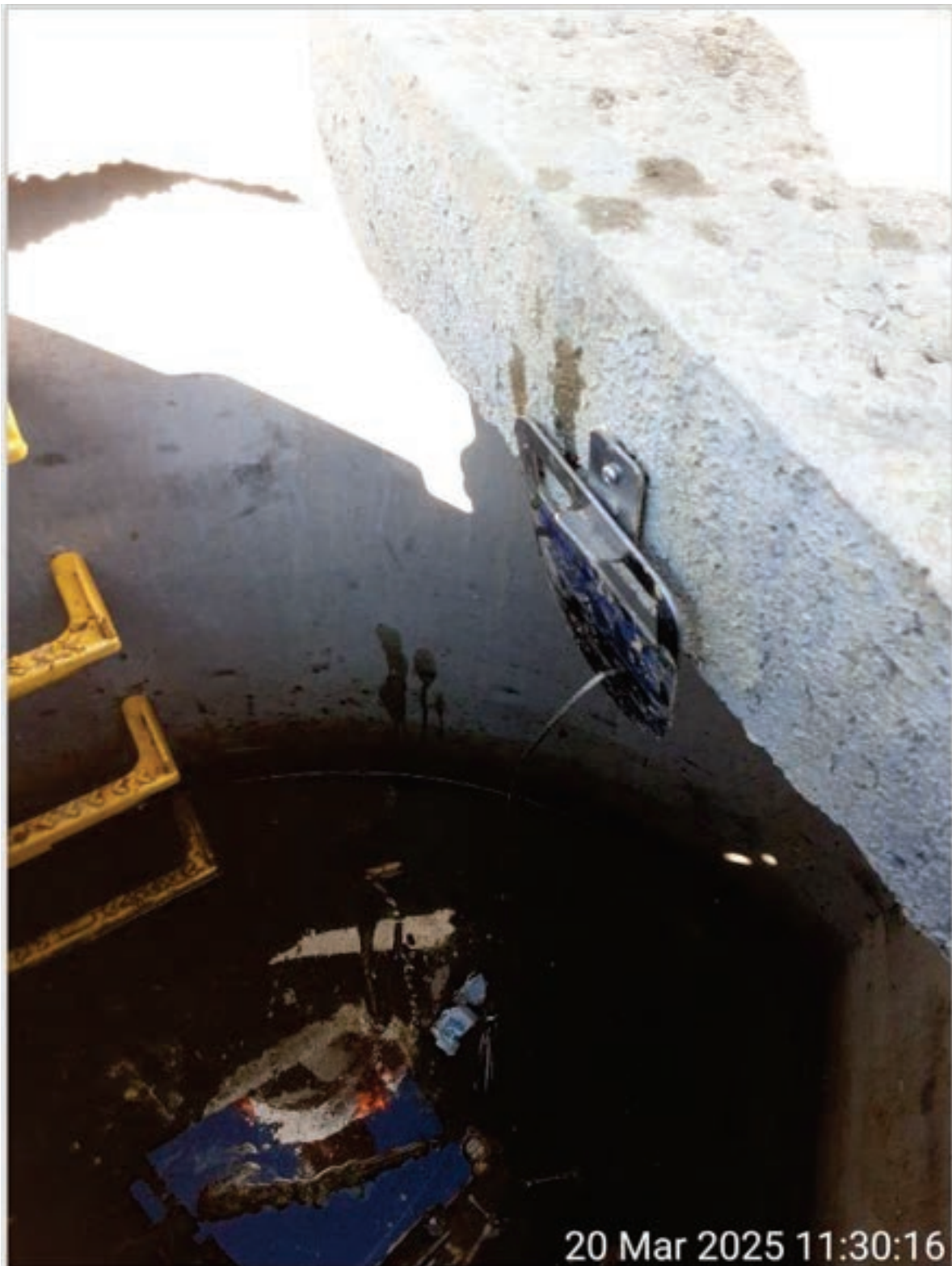
Photo 11 – Hydro-brake pull handle
