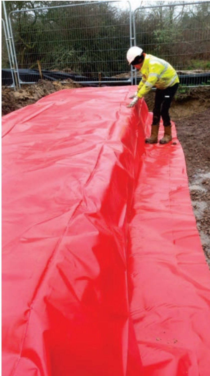
Photo 16 – Culvert A membrane installation
