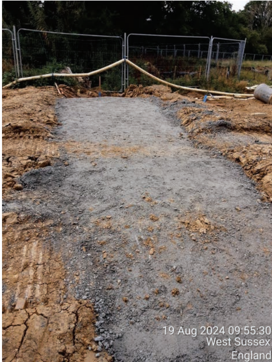
Photo 22 – Culvert C installation
