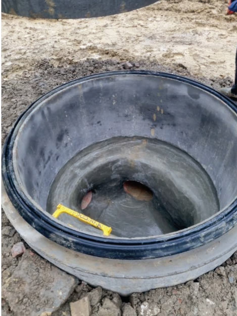
Photo 25 – Base of manhole S28
