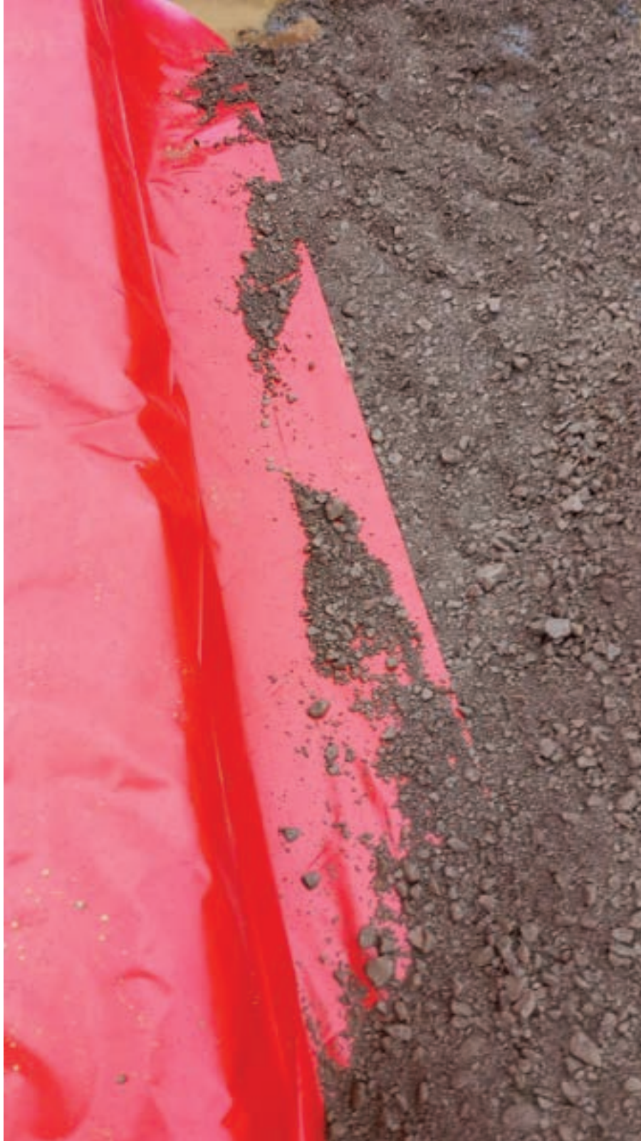
Photo 17 – Culvert A membrane installation
