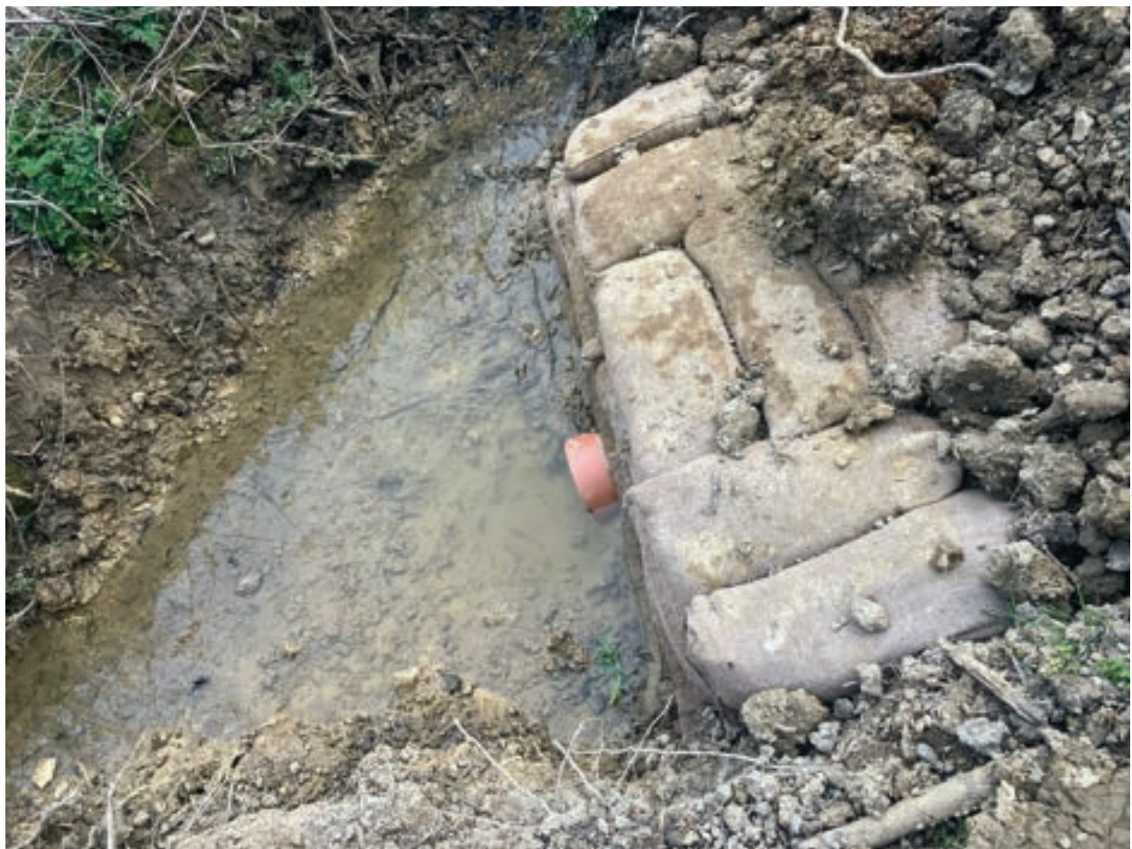
Photo 14 – View of outfall
