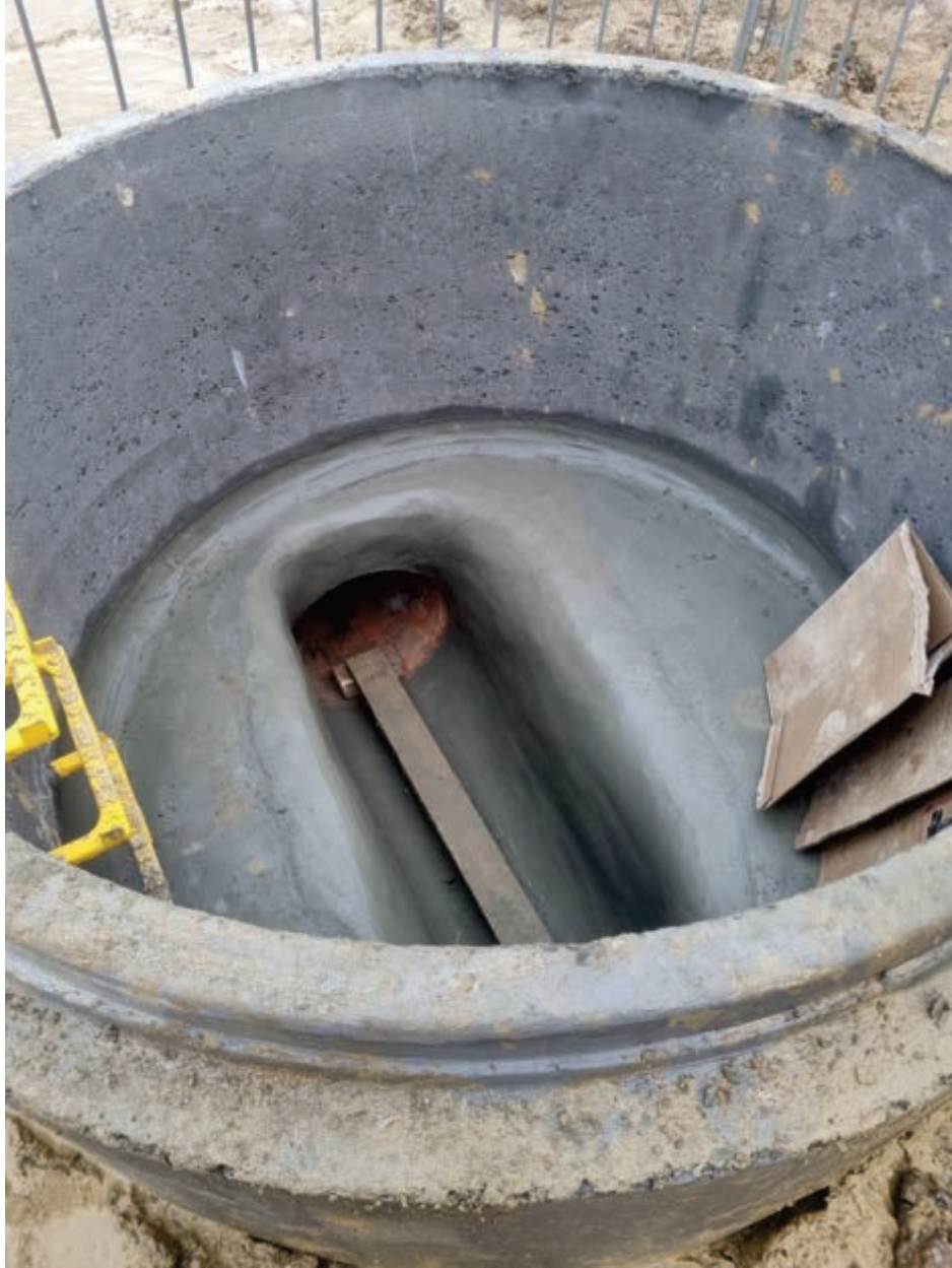
Photo 26 – Base of manhole S29
