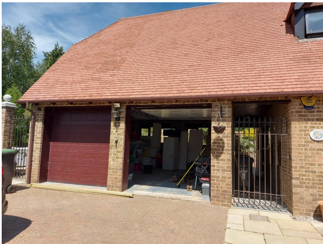
Close up of the existing garage frontage
