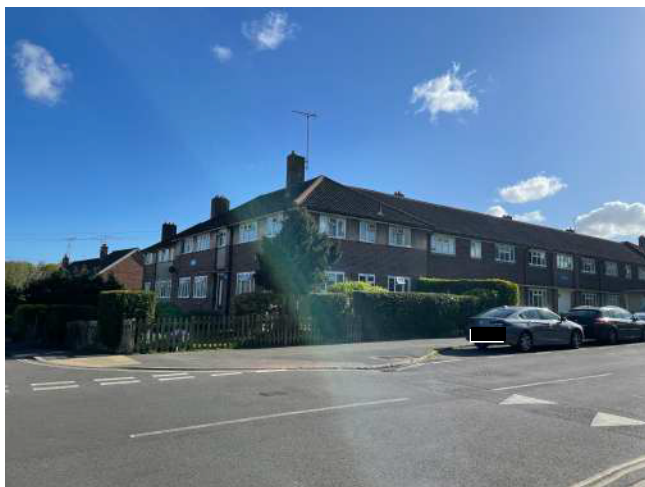
Looking south west from America Lane towards Boston Court on the corner of Boston Road and America Lane.
