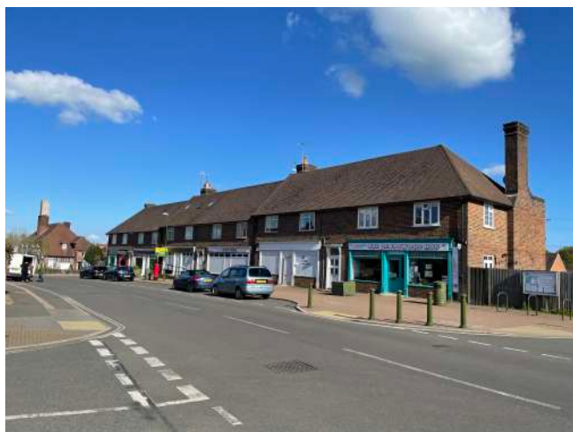
Looking south east towards 34-56 America Lane.
