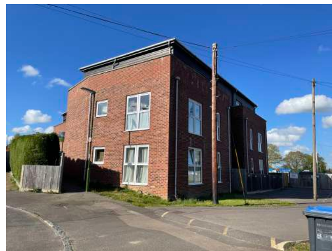
Fenway House - block of 13 flats to south east of Hanbury Football Stadium to south east of Boston Road.
