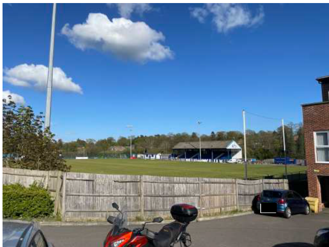
Hanbury Football Stadium to south east of Boston Road.
