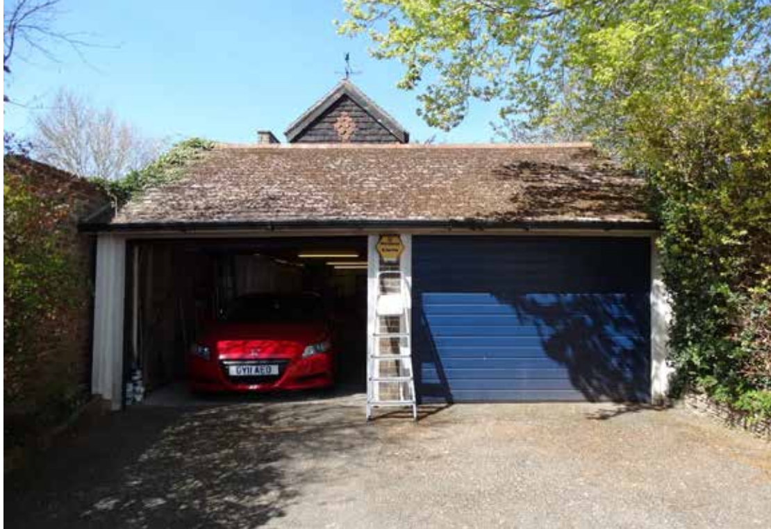
The Garage Frontage
